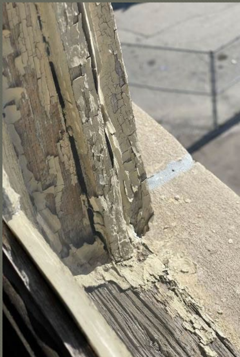
Existing window deterioration
