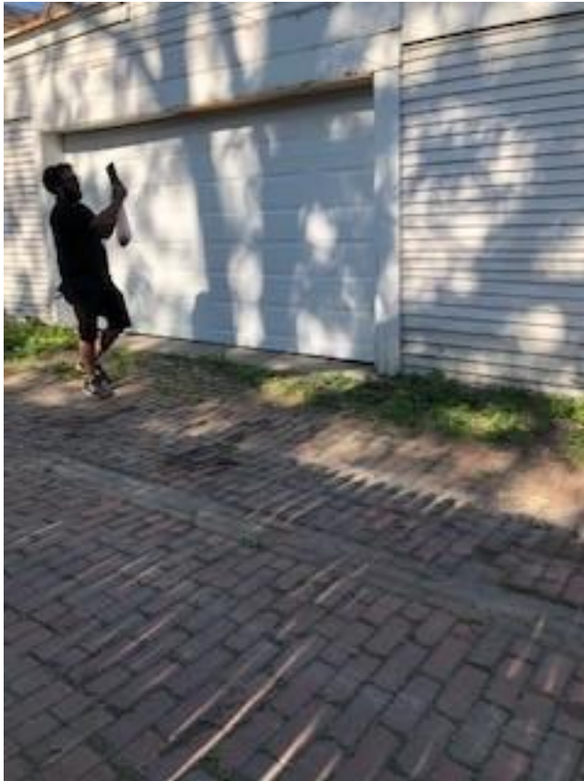
Garage overhead door as completed.
