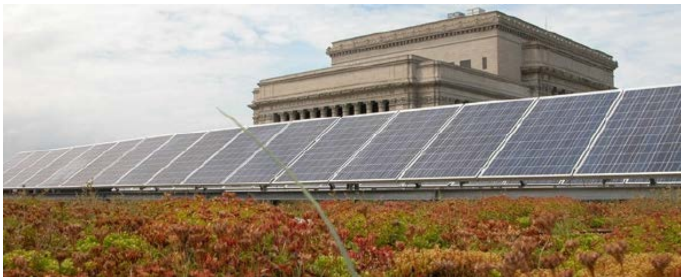
1 Solar Panels on Milwaukee's Central Library
