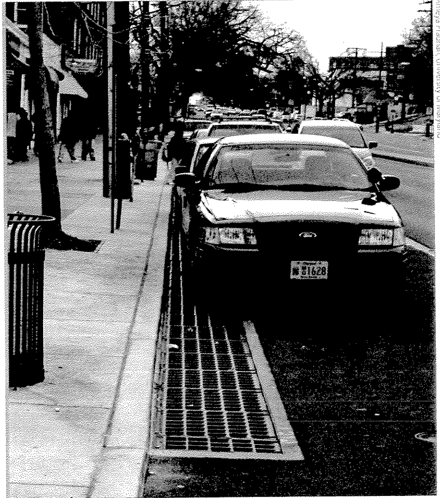
A gutter filter cleanses runoff before sending water to the stormdrain.
