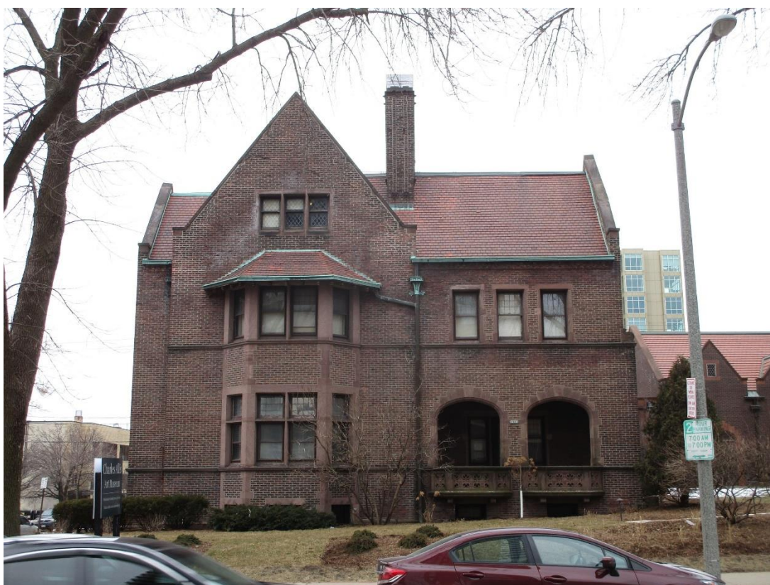
Image 3: Charles Allis Art Museum: East Elevation (View from Prospect Avenue)
