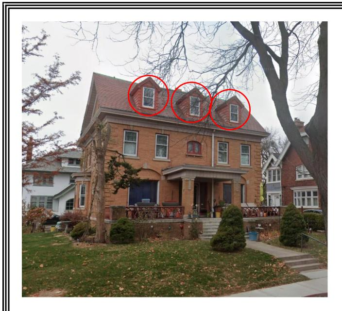
Fiber cement siding on these dormers to be replaced with cedar lap siding and trim
