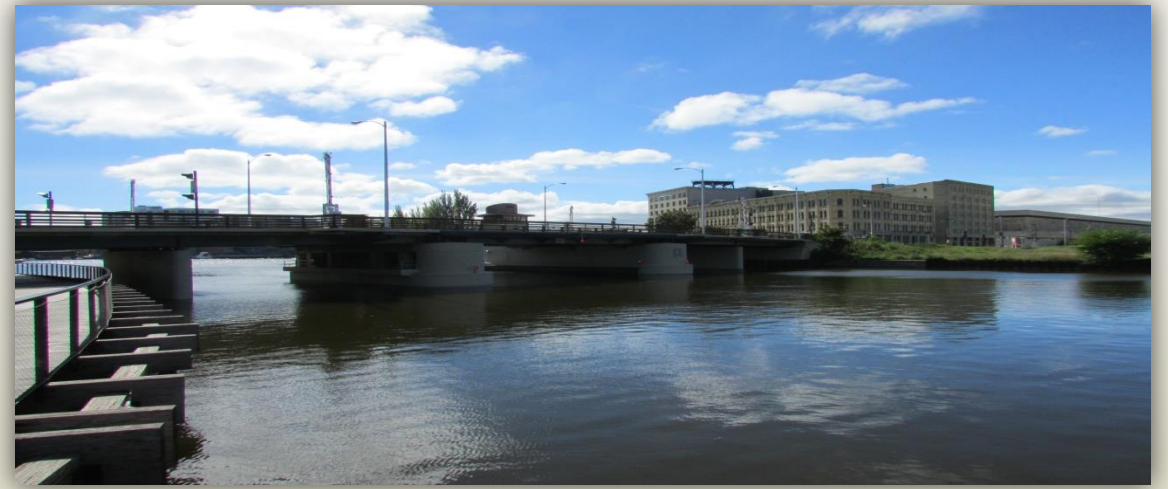
St. Paul Ave. Bridge re-opened on June 11, 2014
