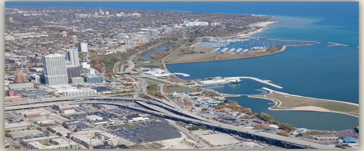
Milwaukee Gateway Project
