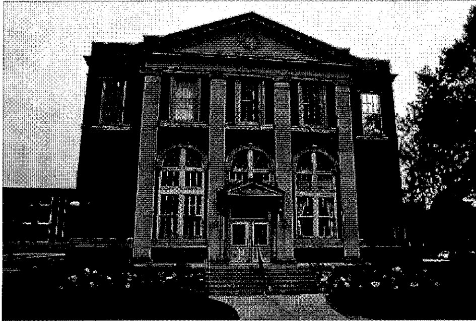
Photo 1 – West elevation of Library
