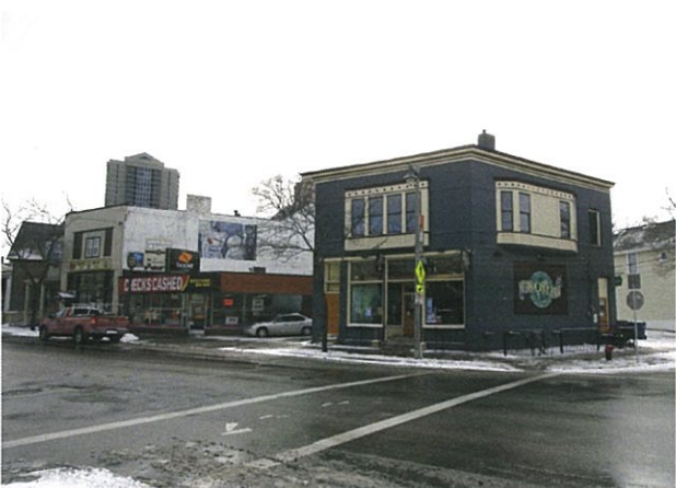
STREETSCAPE PHOTOGRAPH ACROSS BRADY STREET - SOUTHEAST CORNER
