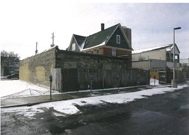
ADJACENT PROPERTY PHOTOGRAPH JIMMY JOHN'S - NORTH SIDE OF EXISTING BUILDING
