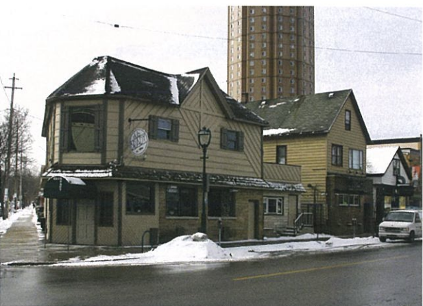
STREETSCAPE PHOTOGRAPH ACROSS BRADY STREET - SOUTHWEST CORNER
