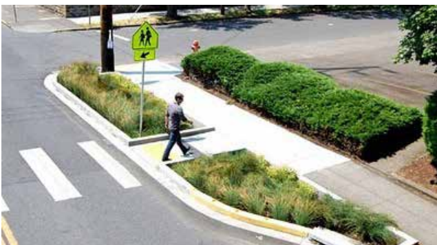
curb bump outs with drainage gardens
