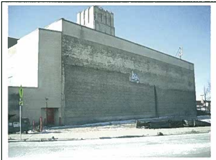
Pic #3 - Looking North West
