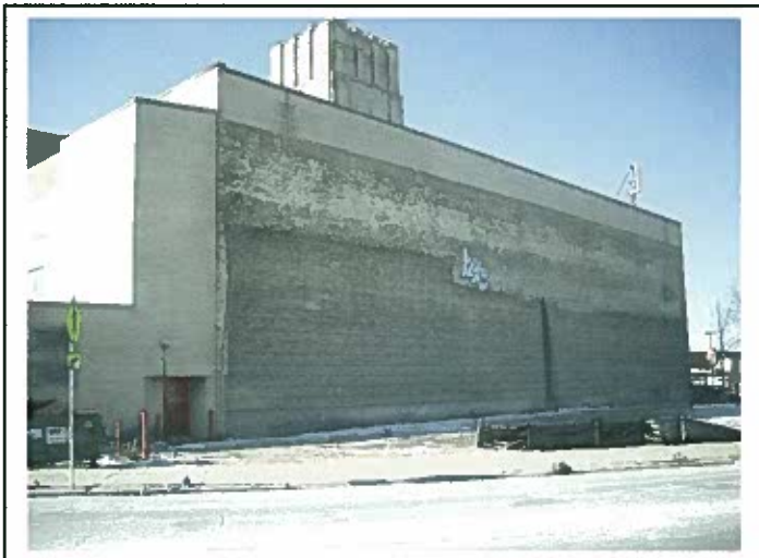
Pic #3 - Looking North West
