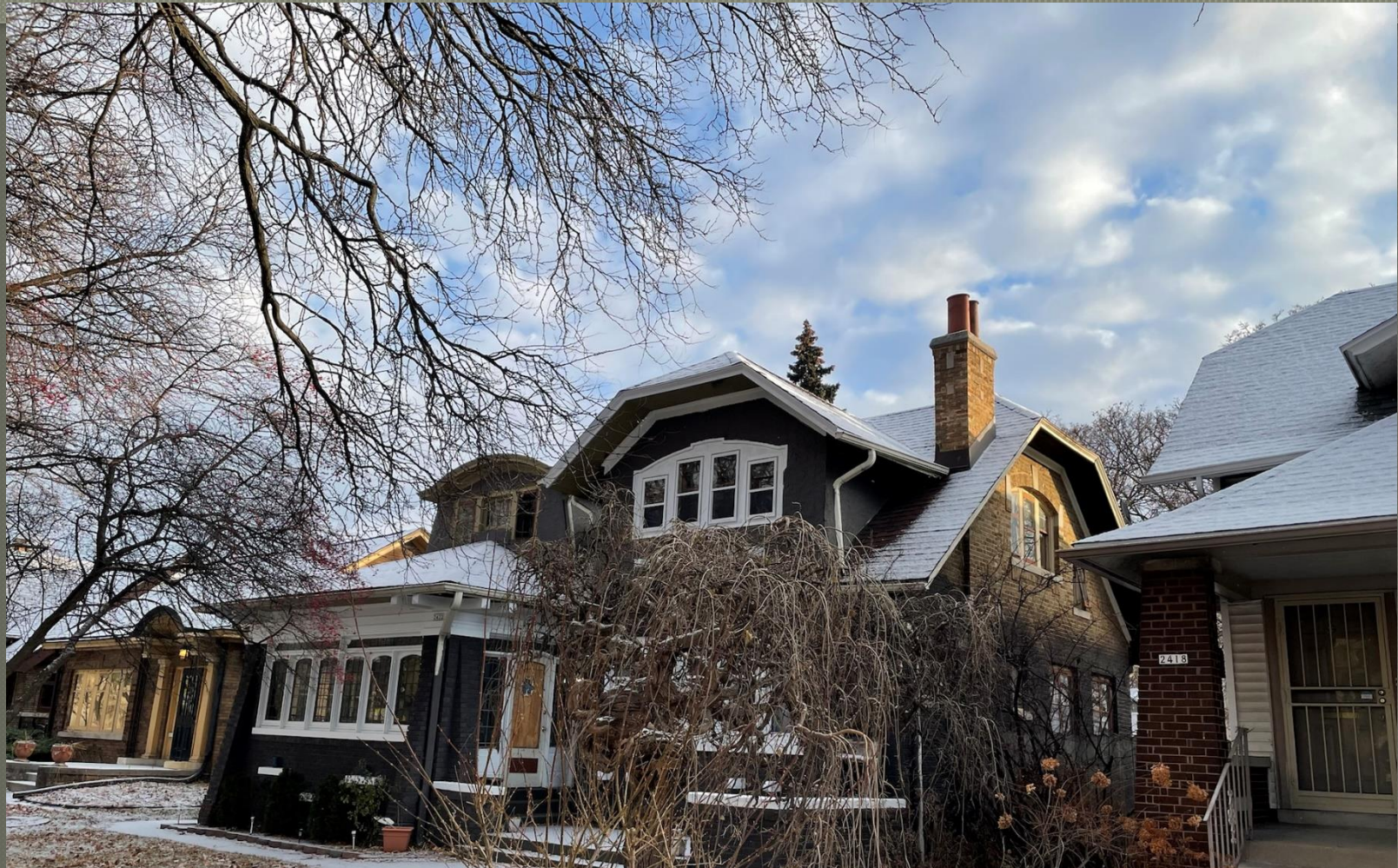
Staining in progress. Original brick visible at upper right
