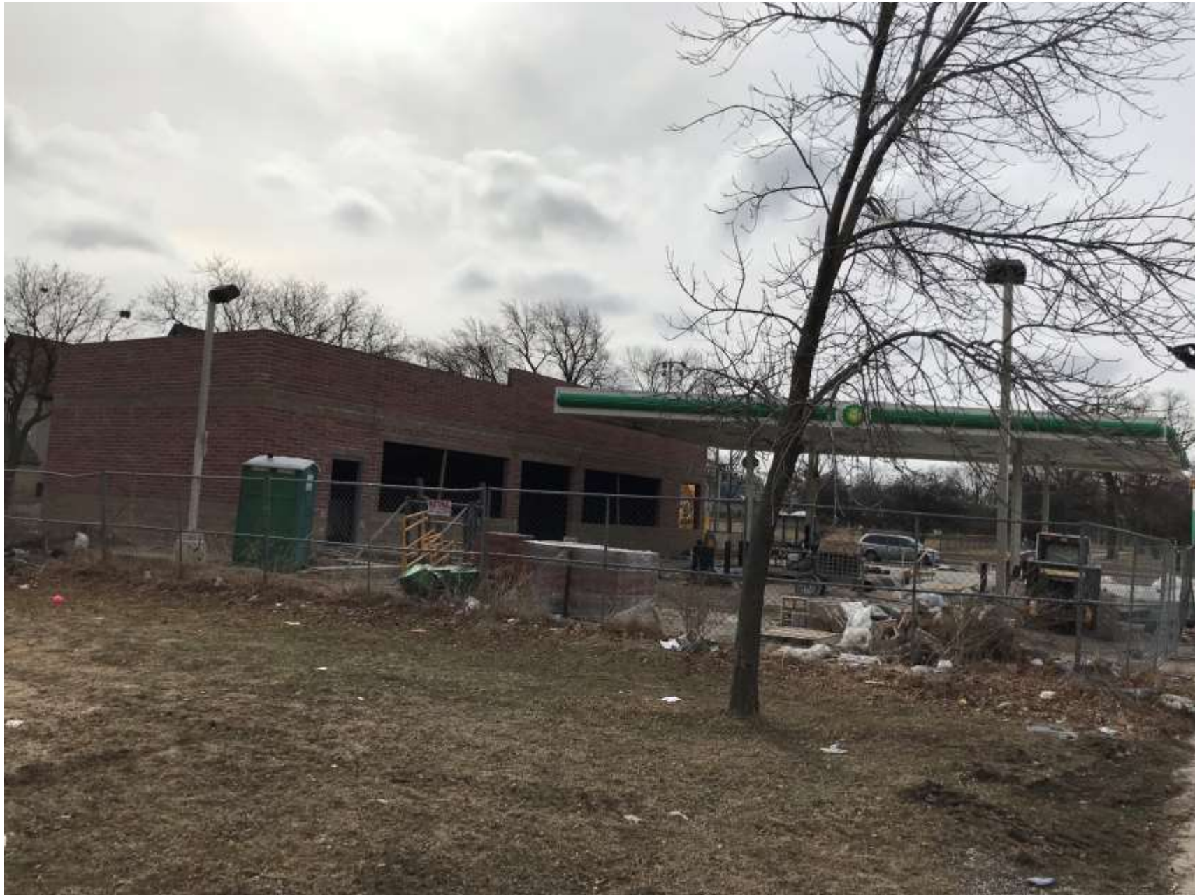
Construction progress photo
