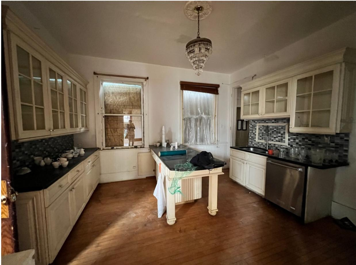
S7 - 2904 W State St Kitchen, facing north. Kitchen cupboards and counter tops are in good shape and are reusable. Two windows are missing storms and missing glazing with some deteriorated wood. Plaster/drywall mostly intact with area of texture imperfections, wood floors are scratched and areas of patches
