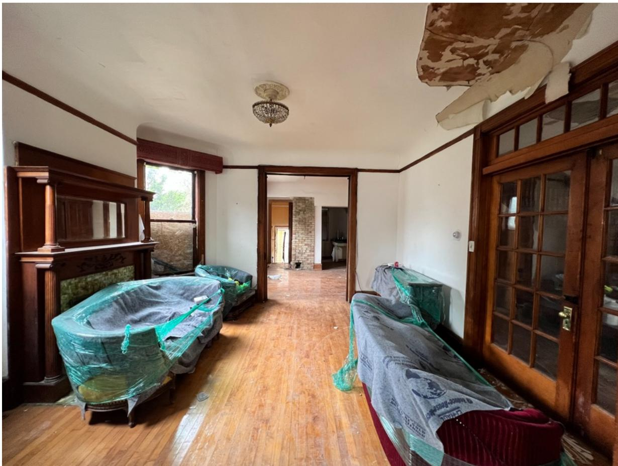
S3 - 2904 W State St Living Room, facing north. A large chunk of ceiling plaster/drywall is missing due to water damage. Wood floors are scratched. Fireplace mantel is intact but some tile is missing.
