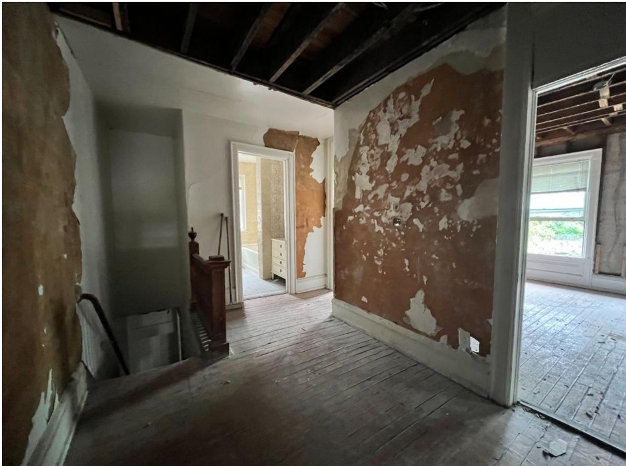
S28 - 2902 W State St top of Grand Staircase, facing north. Missing and cracking drywall/plaster, scratched wood floors, some stairs spindles missing or broken.
