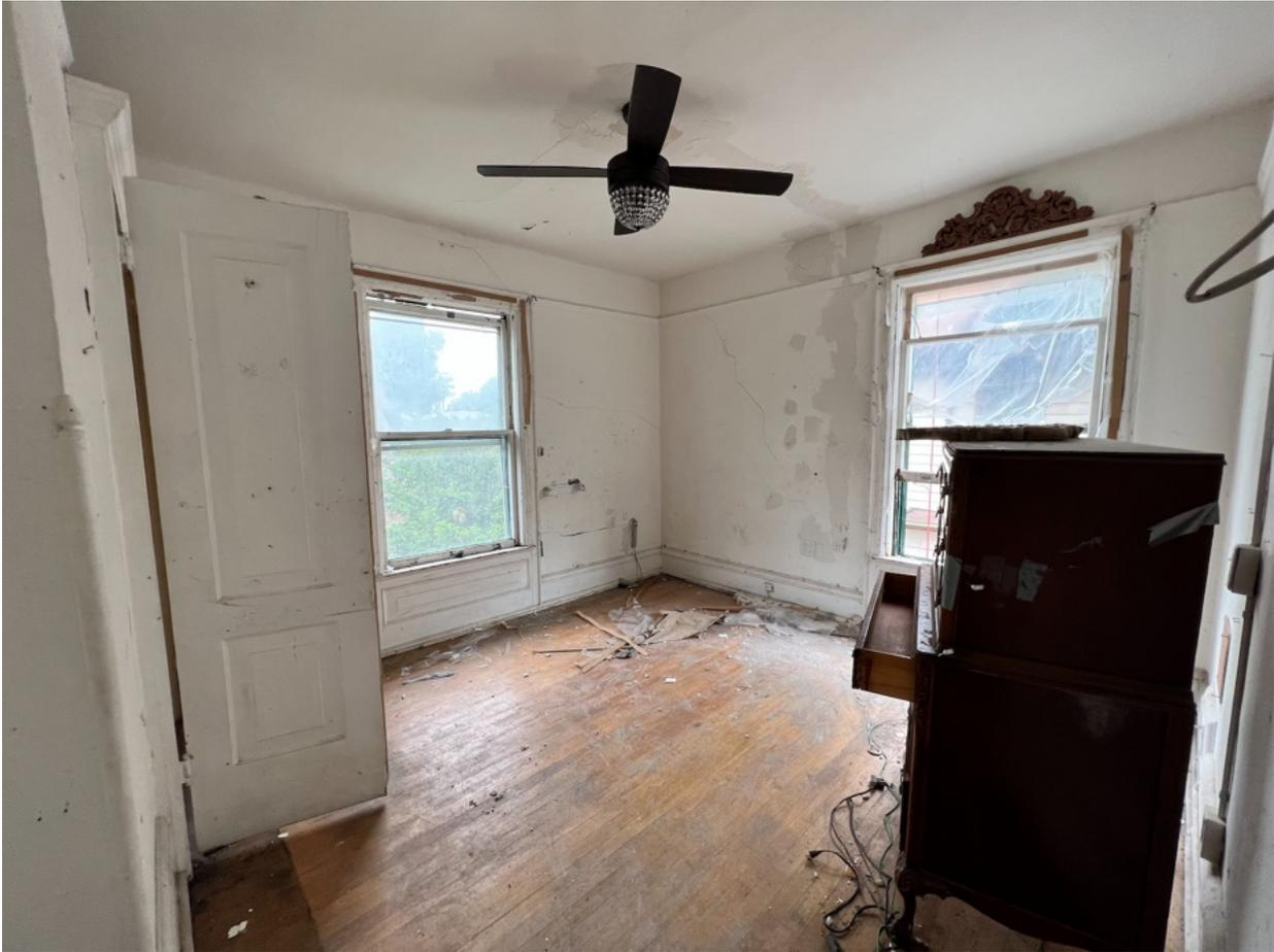
S11 - 2904 W State St Bedroom, facing northwest. Plaster/drywall and wood trim damage throughout. Wood floors are scratched. Windows are missing storms, have broken panes and some rotting wood.
