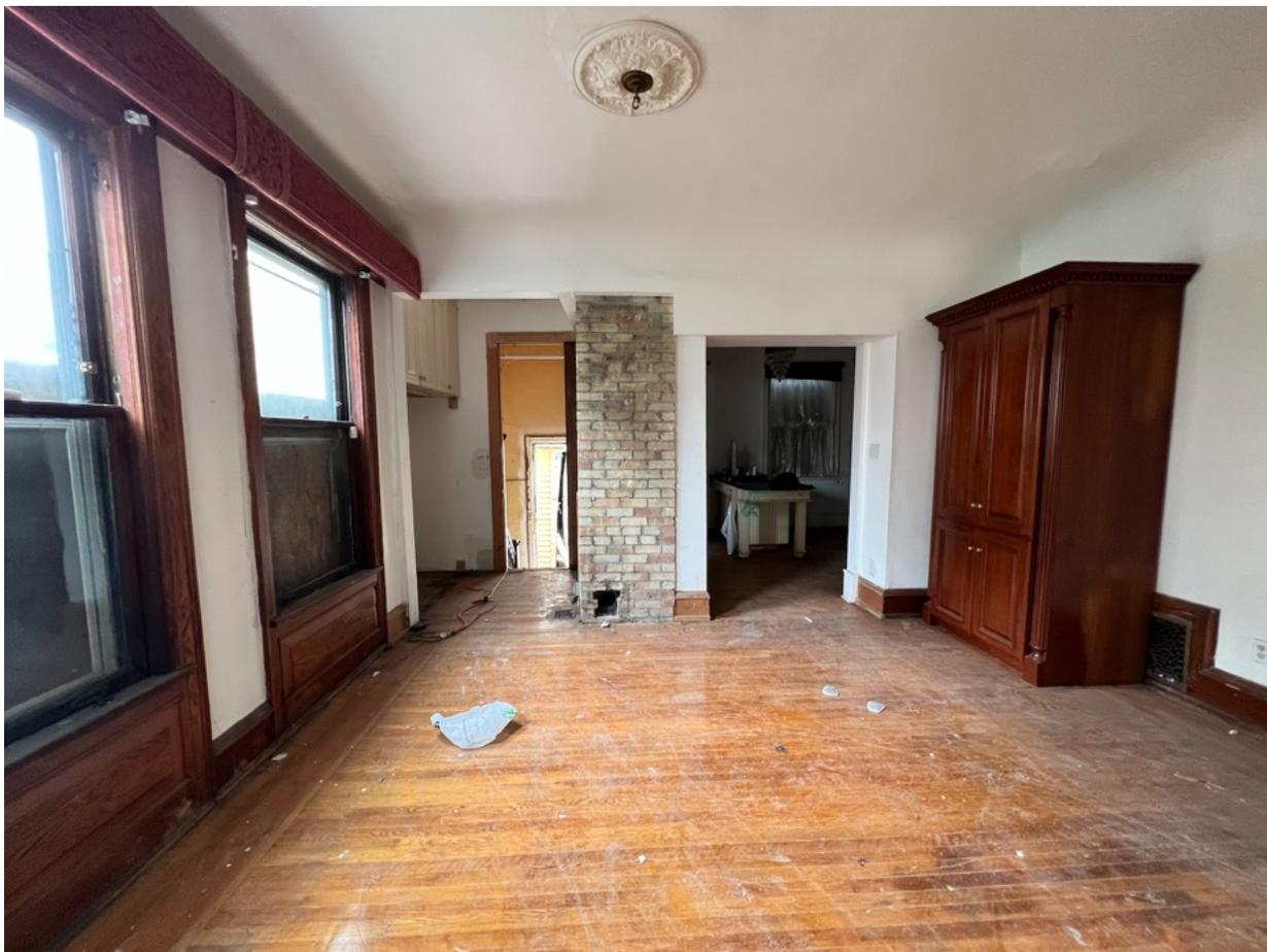
S4 - 2904 W State St Dining Room, facing north. Plaster/drywall is mostly intact, wood floors are scratched, chimney brick is exposed, two windows are missing storms. Windows are missing glazing and have some deteriorated wood. No light fixture.
