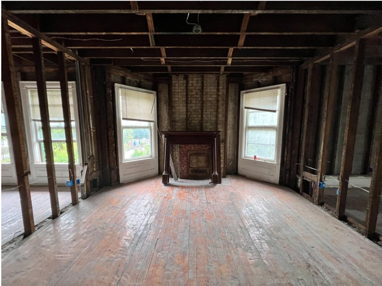
S31 - 2902 W State St second Bedroom, facing east. Plaster/drywall and wood trim damaged/missing throughout. Wood floors are scratched. Windows are missing storms, have broken panes and some rotting wood. fireplace mantel intact but not attached to wall. Fireplace missing some tile.
