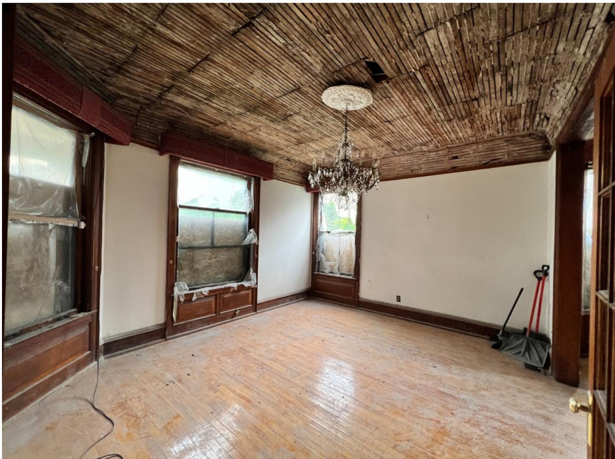
S2 - 2904 W State St Family Room, facing southwest. Majority of the ceiling and wall plaster/drywall is missing/damaged due to water penetration. Hardwood floors are scratched, windows are missing storm windows and have broken window panes and deteriorated/rotting wood frames. Chandelier is broken.
