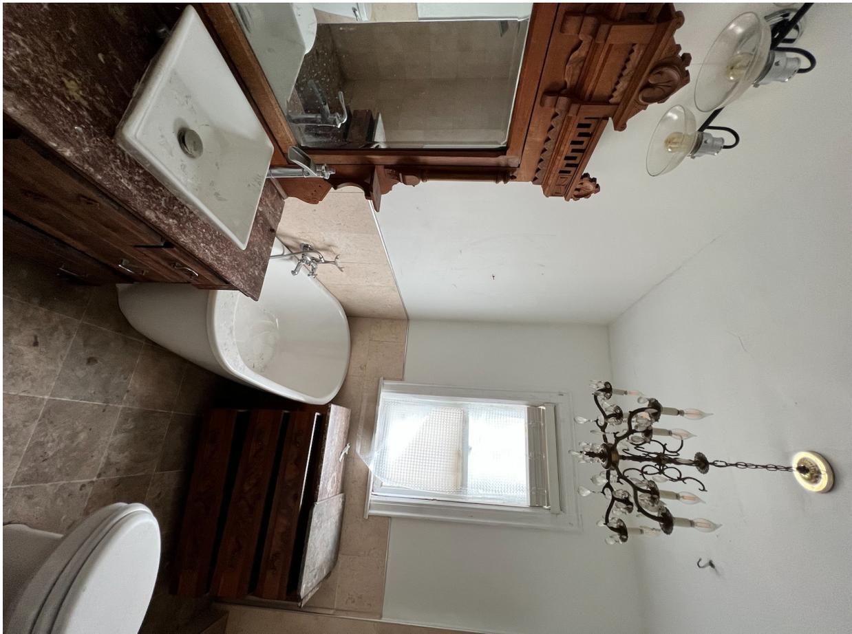
S10 - 2904 W State St upper Bathroom, facing north. Fixtures present but significant wear and tear to vanity, bathtub and toilet. Cracked tile and plaster/drywall throughout.
