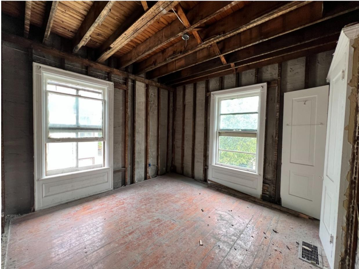
S33 - 2902 W State St fourth Bedroom, facing northeast. Plaster/drywall and wood trim damaged/missing throughout. Wood floors are scratched. Windows are missing storms, have broken panes and some rotting wood.
