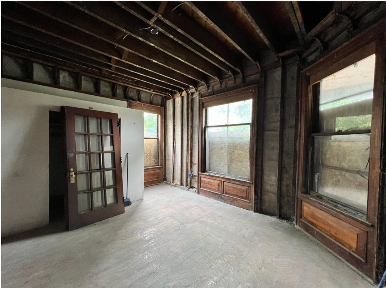
S19 - 2902 W State St Family Room, facing southeast. Majority of the ceiling and wall plaster is missing/damaged due to water penetration. Hardwood floors are scratched, windows are missing storm windows and have broken window panes and deteriorated/rotting wood frames. No working electrical
