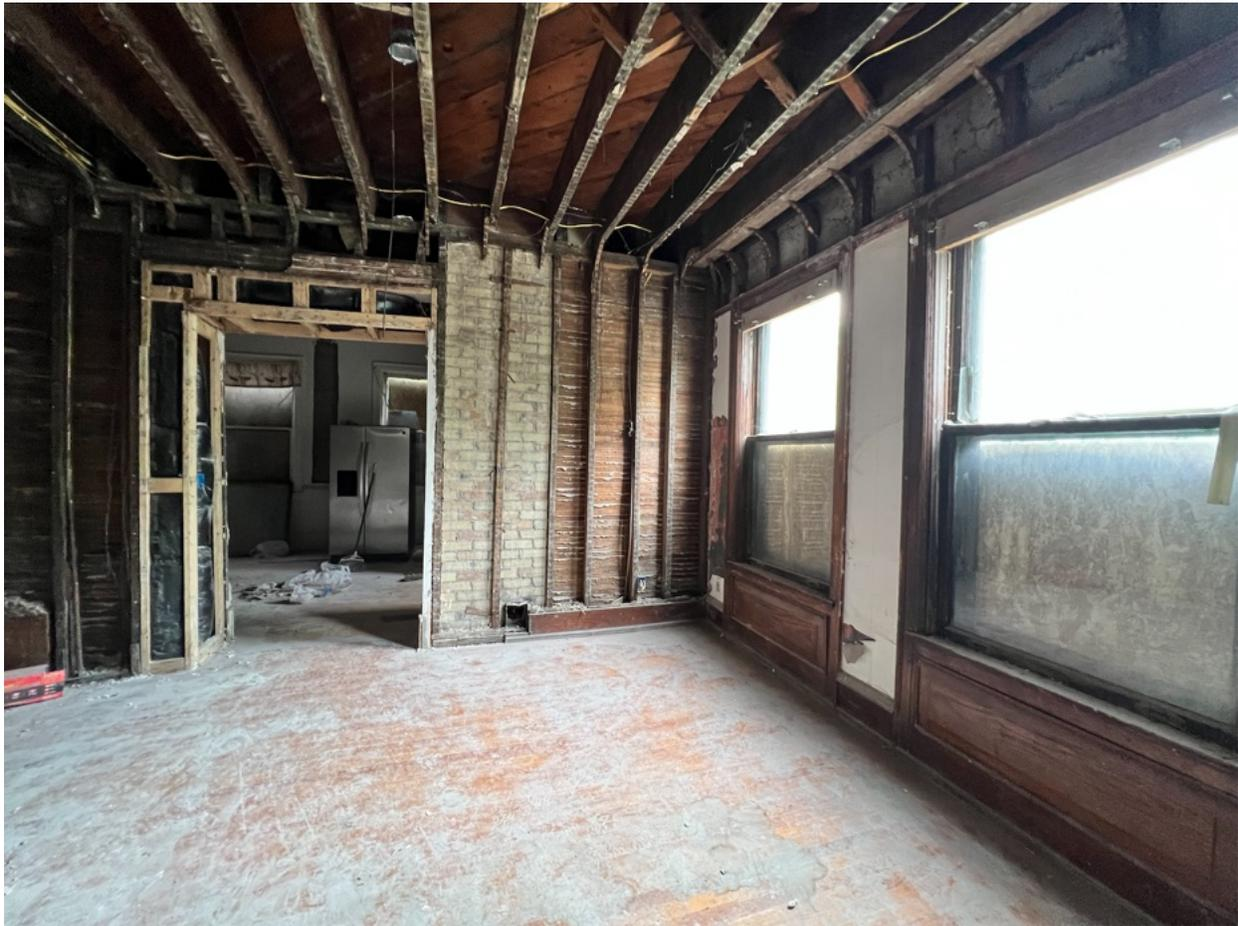
S23 - 2902 W State St Dining Room, facing north into Kitchen. Plaster/drywall is mostly removed, wood floors are scratched, chimney brick is exposed, two windows are missing storms. Windows are missing glazing and have some deteriorated wood.
