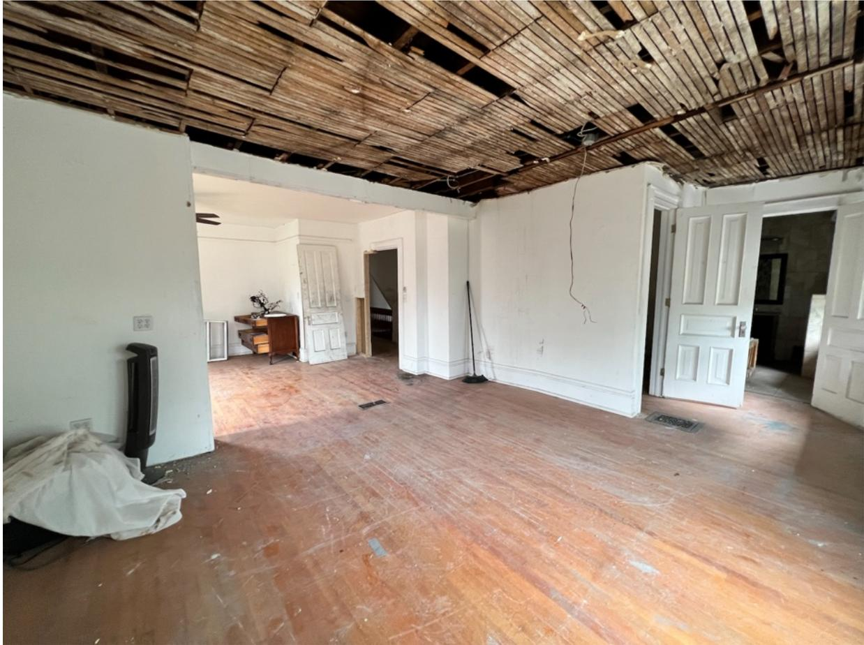
S15 - 2904 W State St third Bedroom, facing northeast. Significant missing plaster/drywall and non-working knob tube wiring. Previously opened up wall to create a master bedroom.
