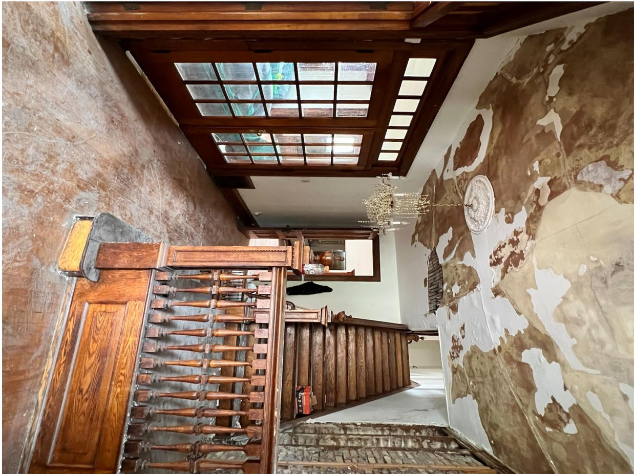
S1 - 2904 W State St Main Entrance, facing north - showing Grand Staircase. The Foyer has suffered from water damage and ceiling drywall/plaster is missing or damaged. The wood floors are damaged, there are missing stair banisters.
