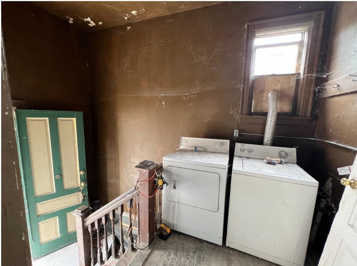
S26 - 2902 W State St back exit, facing east. Plaster/drywall mostly hanging but cracking and crumbling, wood floors are scratched and areas of patches.
