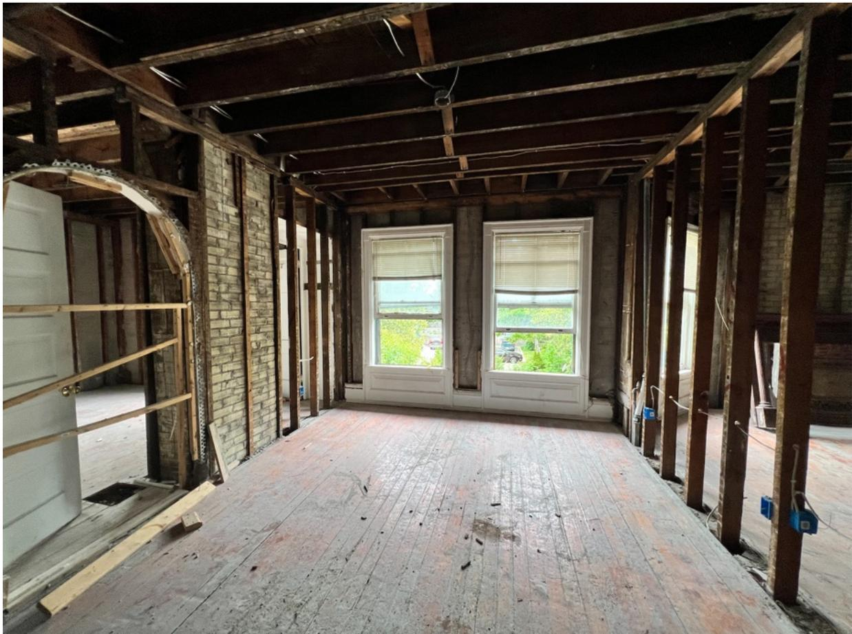
S32 - 2902 W State St third Bedroom, facing east. Plaster/drywall and wood trim damaged/missing throughout. Wood floors are scratched. Windows are missing storms, have broken panes and some rotting wood.
