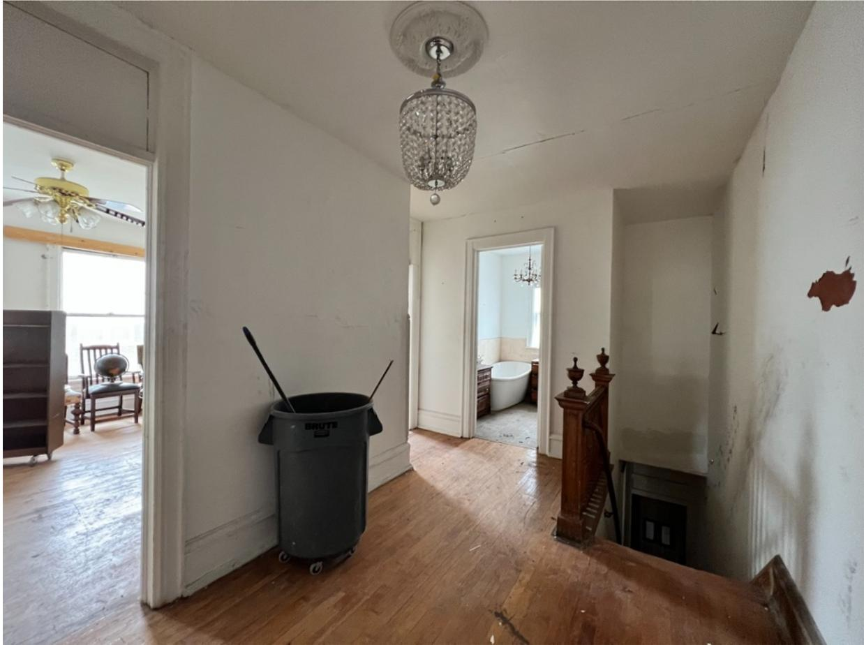
S9 - 2904 W State St top of Grand Staircase, facing north. Missing and cracking drywall/plaster, scratched wood floors, some stairs spindles missing or broken.
