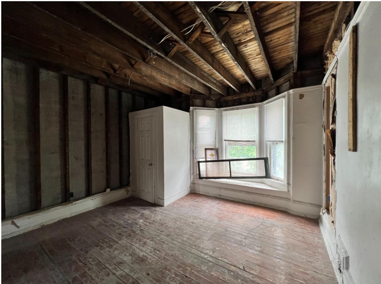
S30 - 2902 W State St Bedroom, facing southeast. Plaster and wood trim damaged/missing throughout. Wood floors are scratched. Windows are missing storms, have broken panes and some rotting wood.
