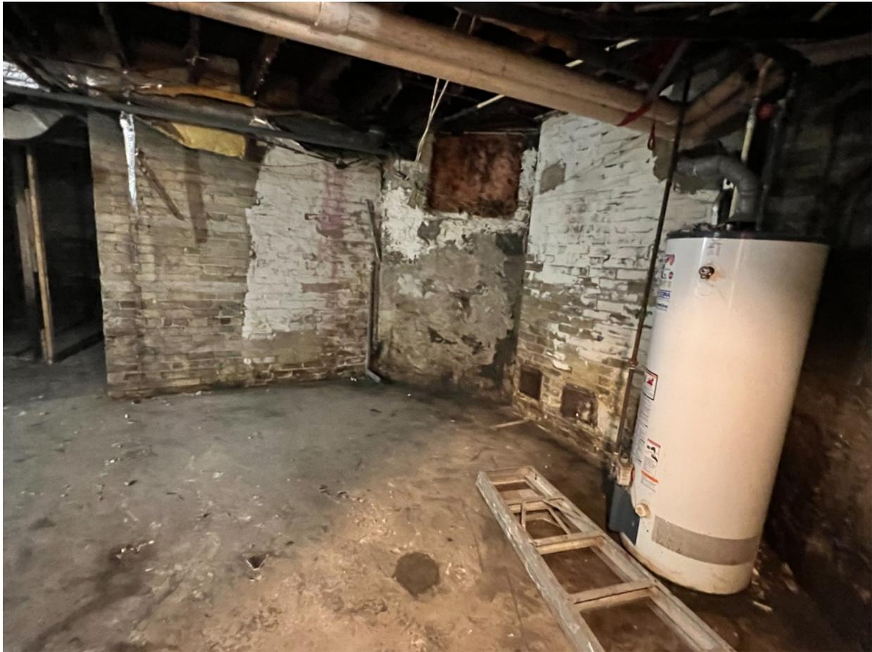
Basement main mechanical room. Showing water damage and brick/stone foundation combination.
