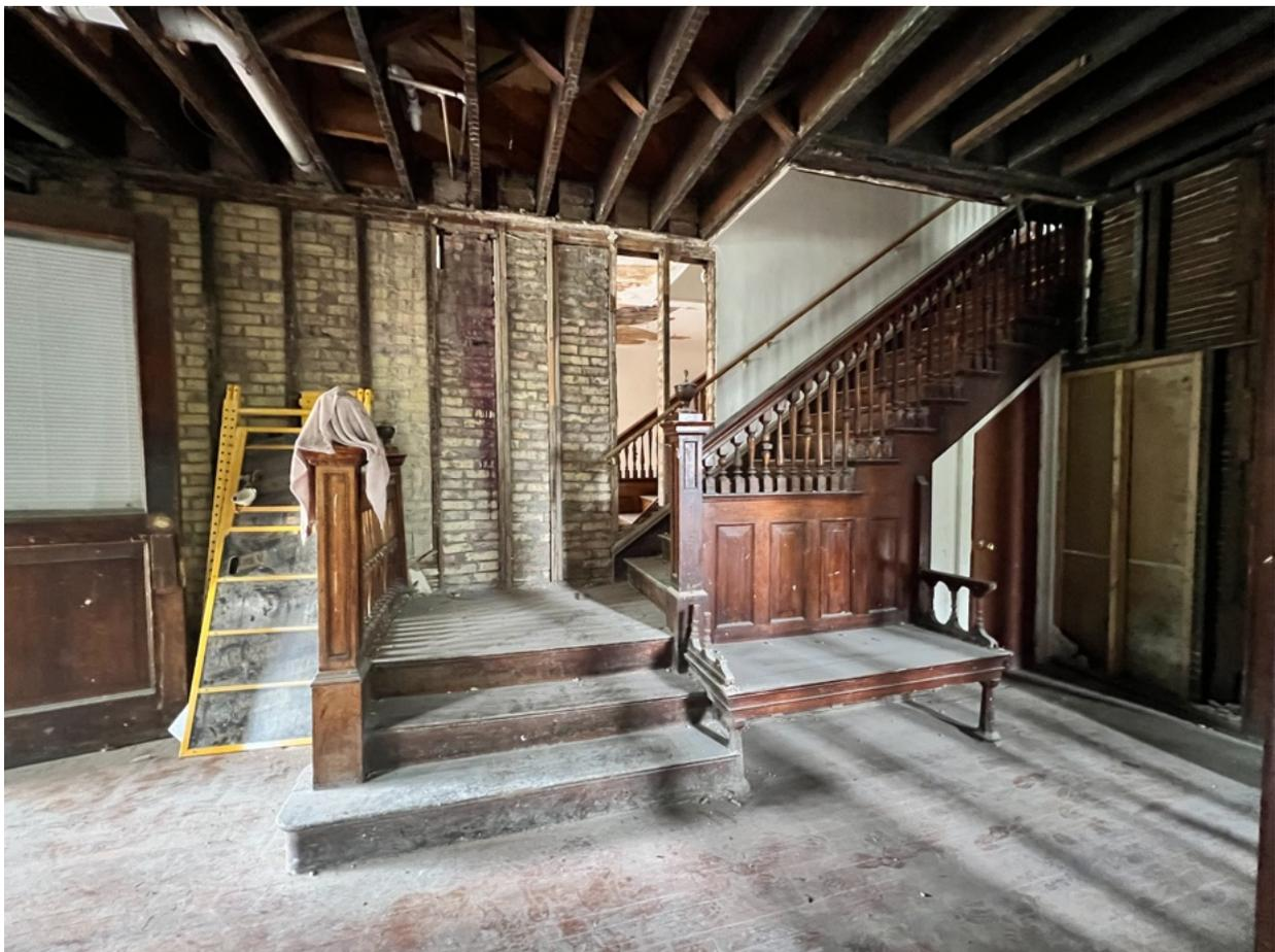
S22 - 2902 W State St Main Entrance and Grand Staircase, facing west. Showing separating wall of masonry (which runs to top floor) and entry bench.
