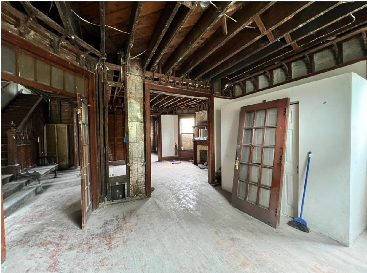
S20 - 2902 W State St Family Room, facing north. Significant missing plaster/drywall and no working electrical. Note cove shaped perimeter.
