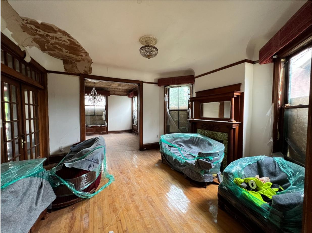
S5 - 2904 W State St Living room facing towards Family Room, facing south. Windows are missing storms and have deteriorated wood frames.
