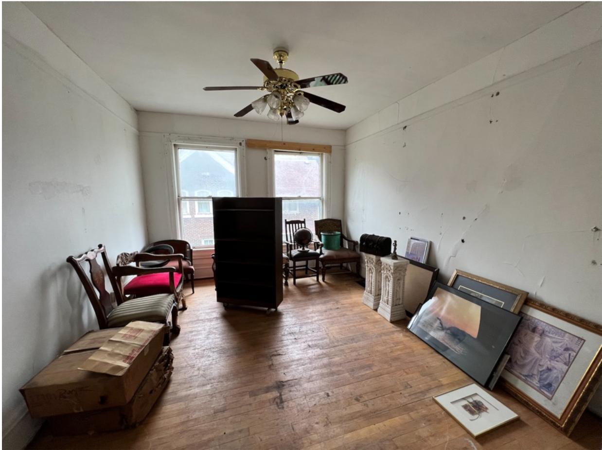
S13 - 2904 W State St second Bedroom, facing west. Plaster/drywall and wood trim damage throughout. Wood floors are scratched. Windows are missing storms, have broken panes and some rotting wood.
