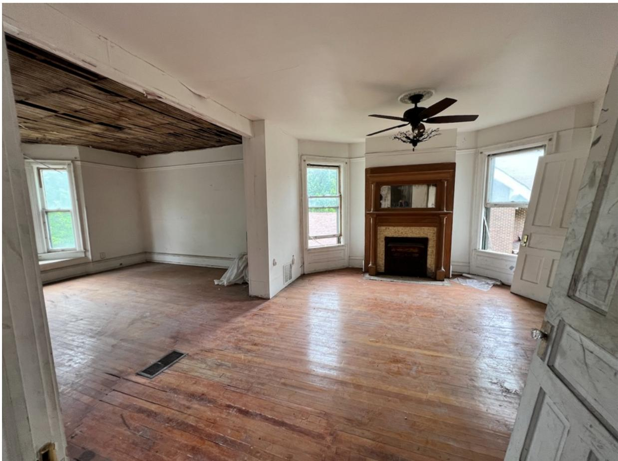
S14 - 2904 W State St third Bedroom, facing southwest. Significant flooring damage and buckling. Plaster/drywall and wood trim damage throughout. Wood floors are scratched. Windows are missing storms, have broken panes and some rotting wood.
