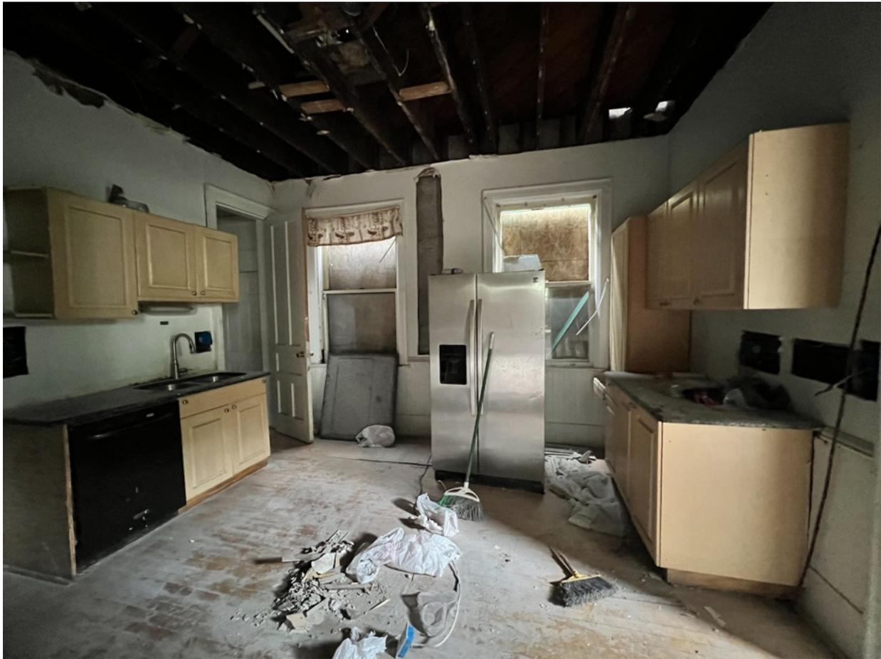
S25 - 2902 W State St Kitchen, facing north. Kitchen cupboards and counter tops are in good shape and are reusable. Two windows are missing storms and missing glazing with some deteriorated wood. Plaster/drywall mostly intact with area of texture imperfections and missing on ceiling, wood floors are scratched with areas of patches.
