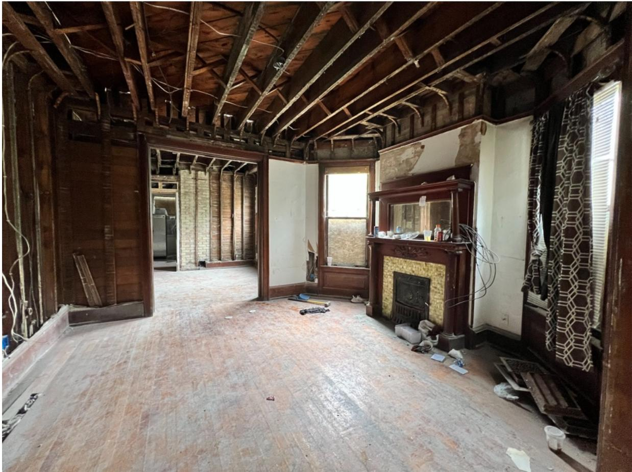
S21 - 2902 W State St Living Room, facing north. All of ceiling plaster/drywall is missing due to water damage. Wood floors are scratched. fireplace mantel is intact but some tile is missing. Windows are missing storms and have deteriorated wood frames.
