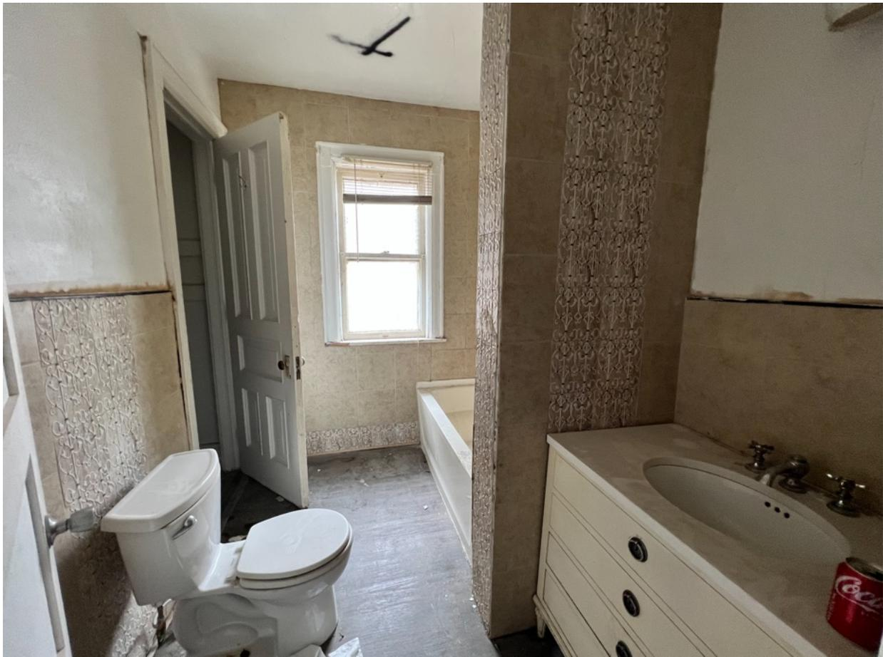
S34 - 2902 W State St upstairs Bathroom, facing north. LVP broken and scratched, vanity, toilet and tub all have wear and tear, tile along wall missing grout and cracked in areas. Window missing some wood framing. Drywall/plaster holes.
