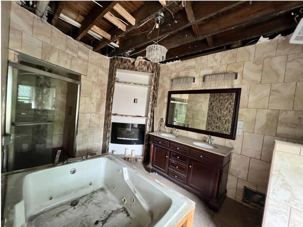
S17 - 2904 W State St Master Bathroom, facing northeast. Significant amount of drywall/plaster missing from ceiling. Tile among walls and floor are cracked. Large tub damaged glazing and inoperable jets, vanity has a decent amount of wear and tear, electric fireplace inoperable, shower tiles damaged.
