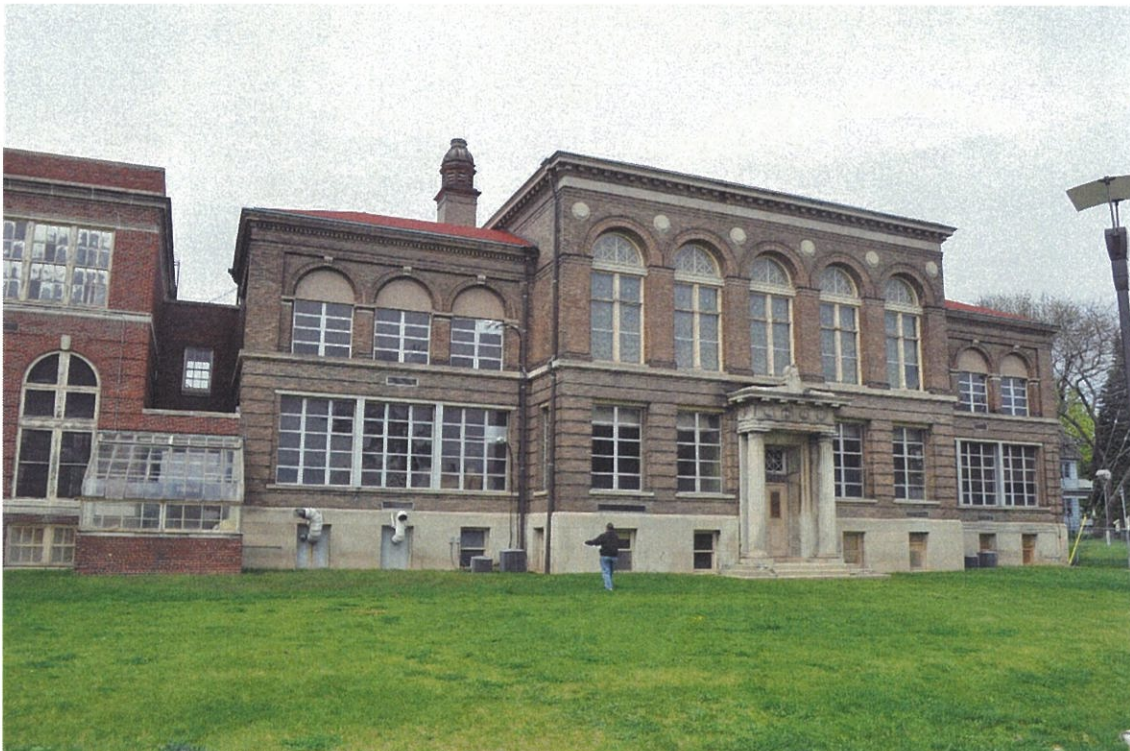
Photo 4 – South elevation of Albrecht Hall
