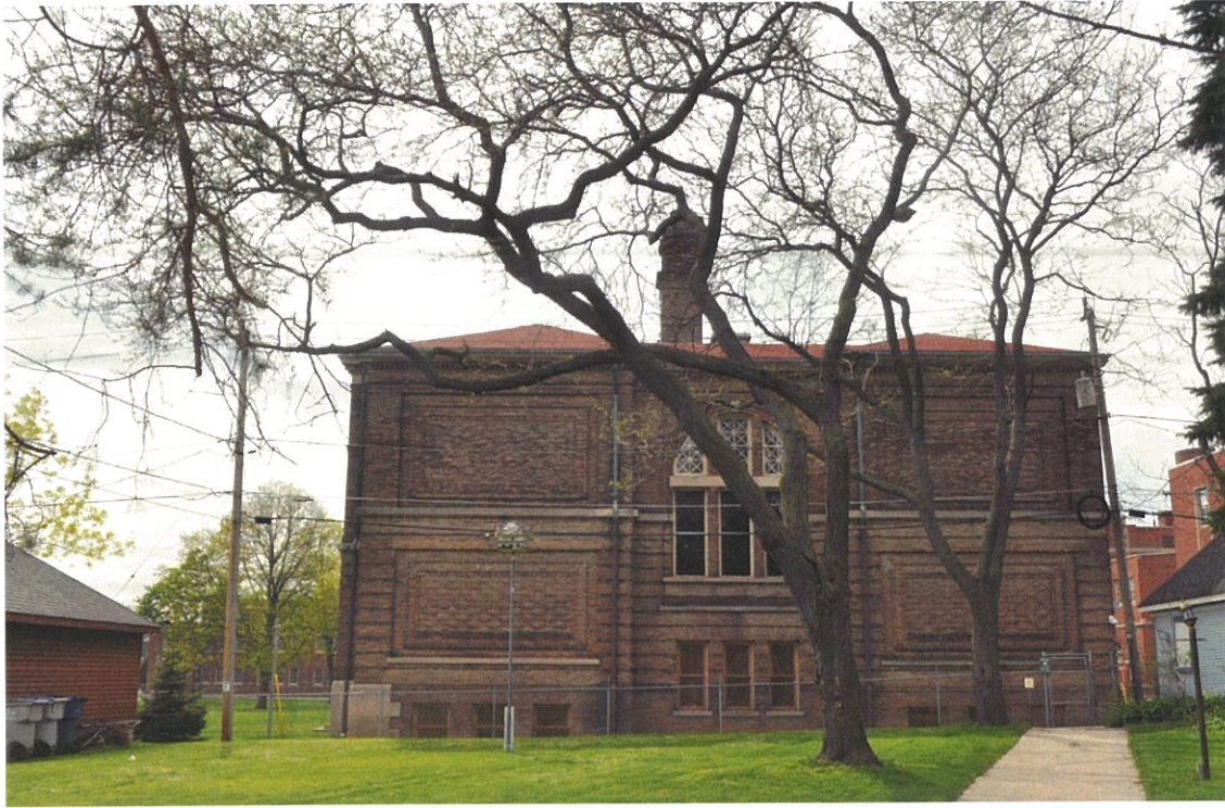
Photo 9 – East elevation of Albrecht Hall
