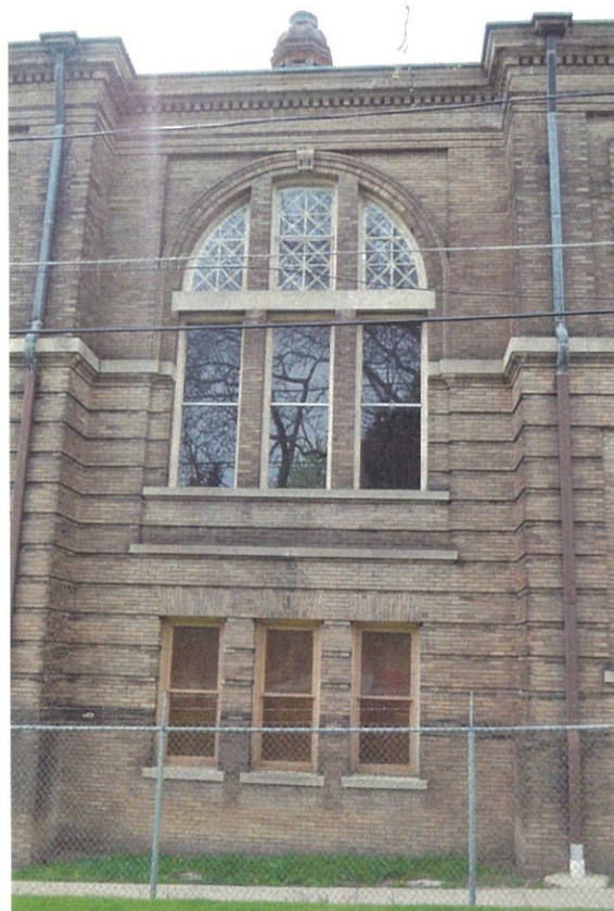
Photo 10 - Window detail on the east elevation of Albrecht Hall
