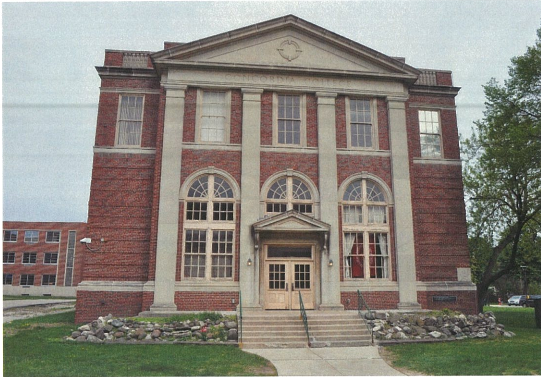
Photo 1 – West elevation of Library
