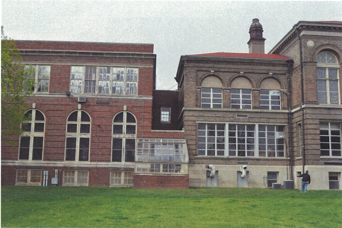
Photo 3 – South elevation of connection between Library and Albrecht Hall
