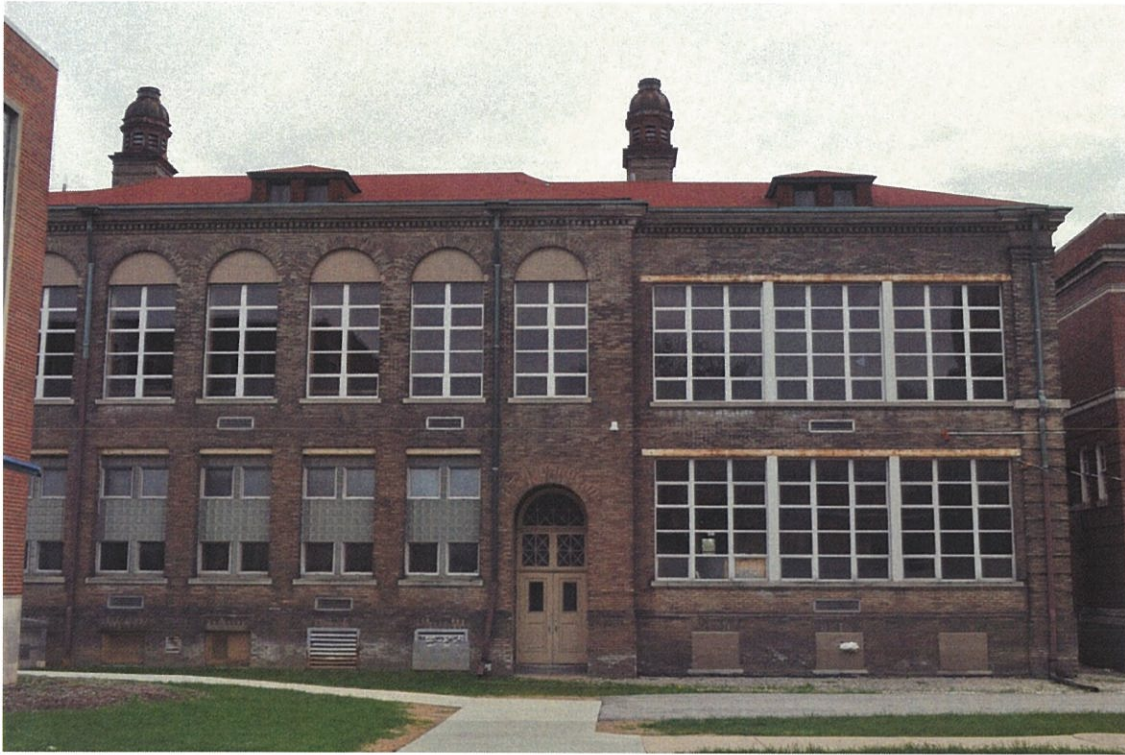
Photo 11 - North elevation of Albrecht Hall
