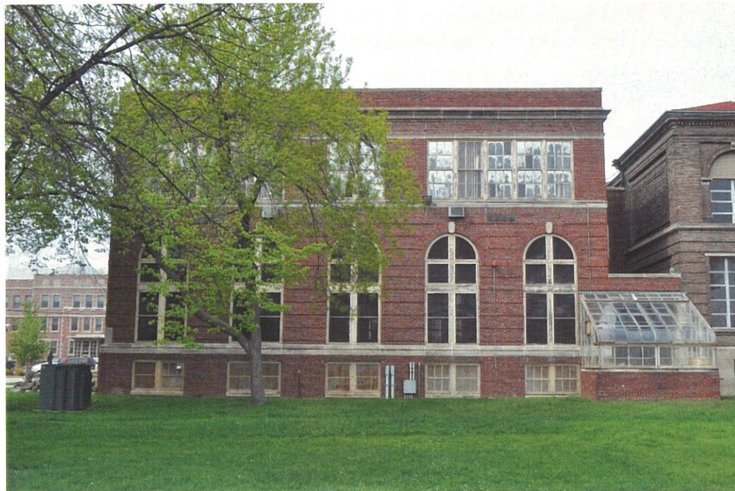
Photo 2 - South elevation of Library
