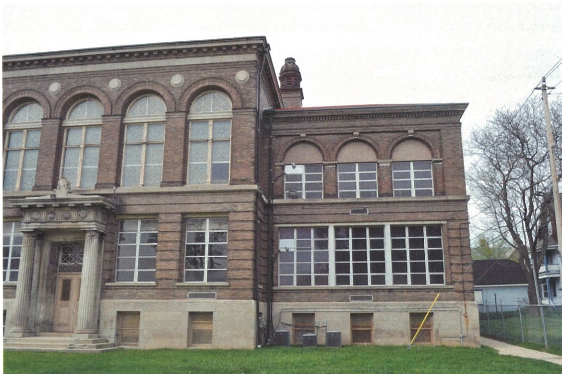
Photo 6 – Windows on south elevation of Albrecht Hall
