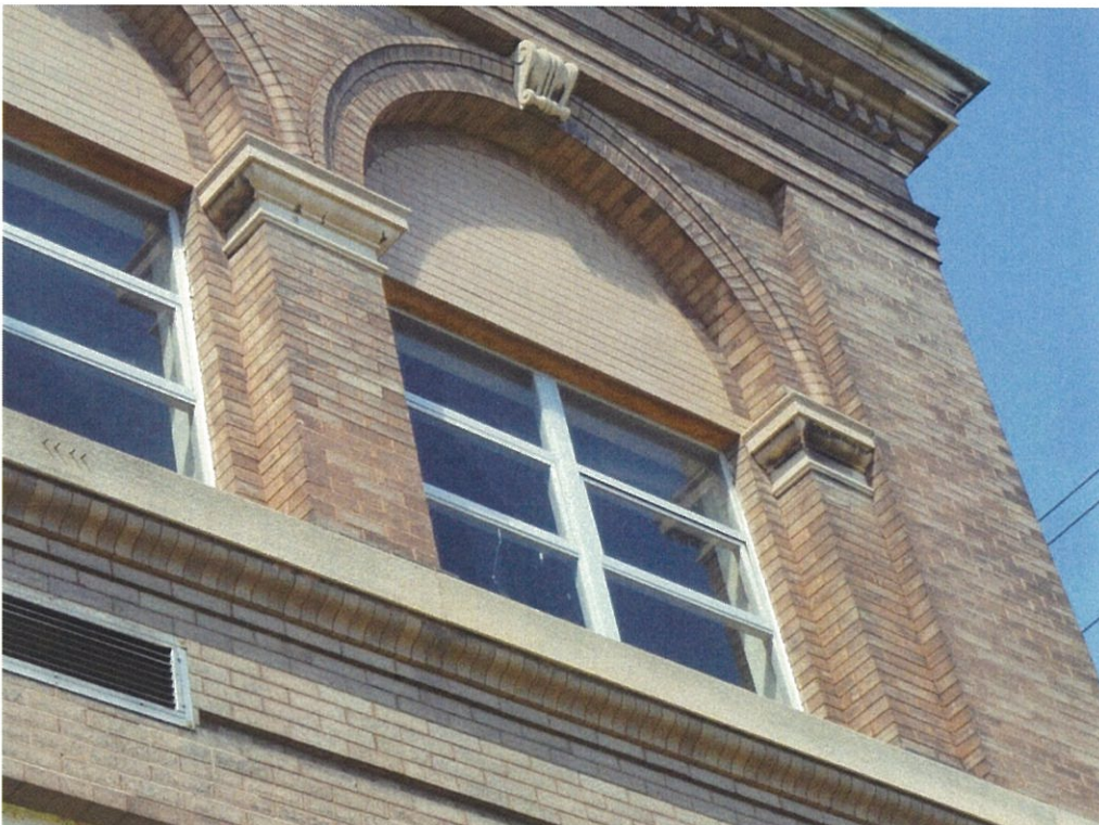
Photo 8 - Detail of window on east end of south facade
