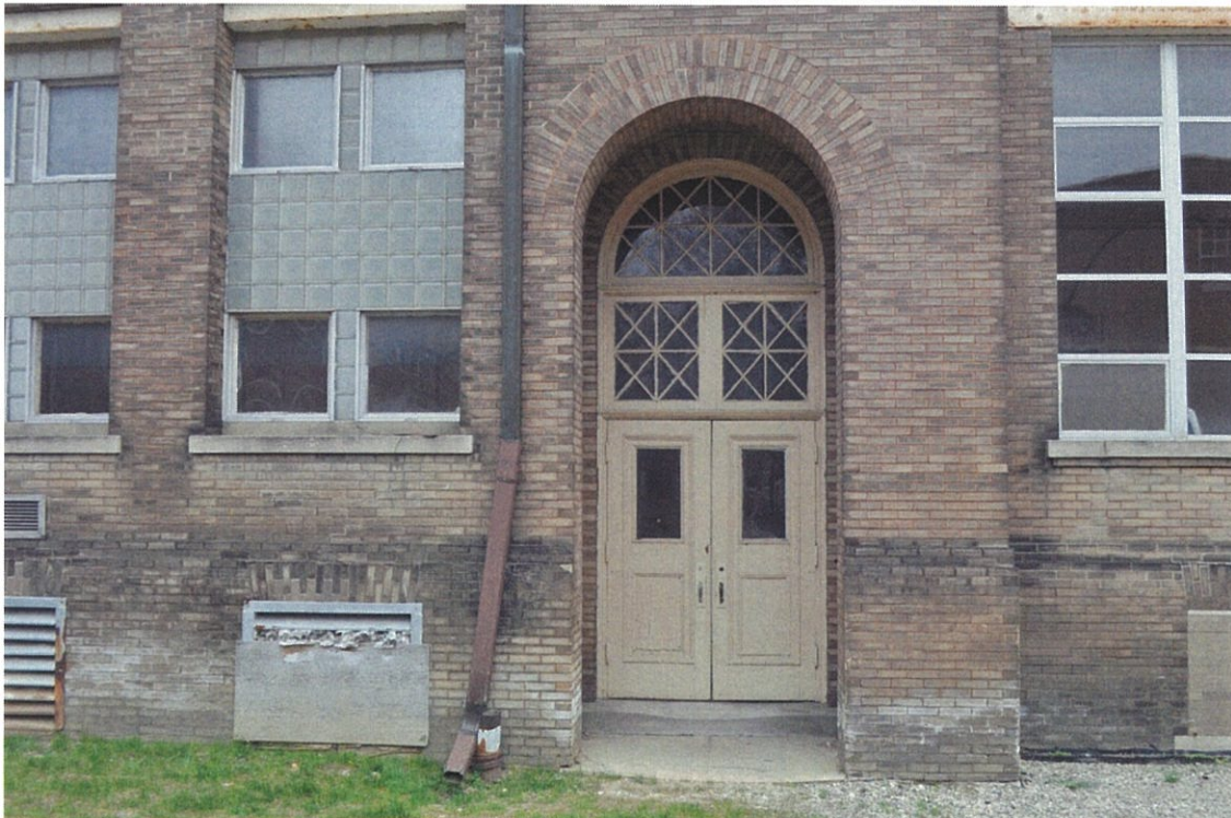
Photo 12 - Archway entrance on north elevation of Albrecht Hall
