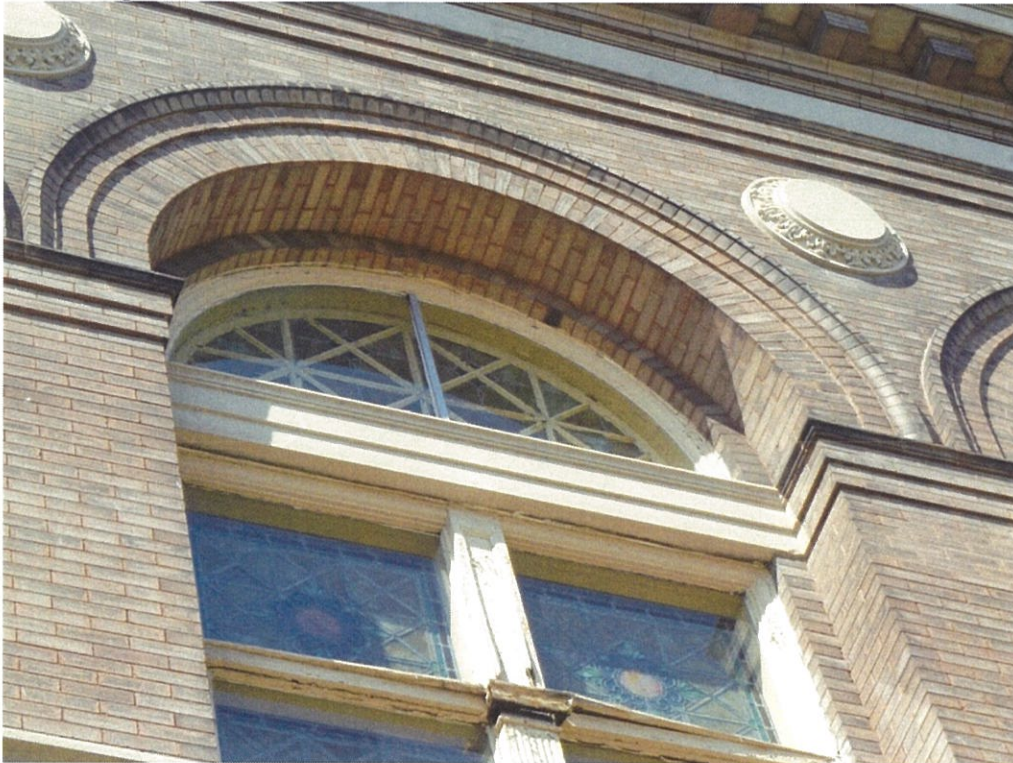
Photo 7- Close-up of central window detailing on south facade
