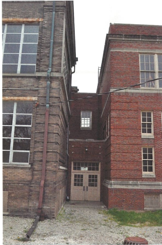
Photo 13 - West elevation of connection between Albrecht Hall and Library
