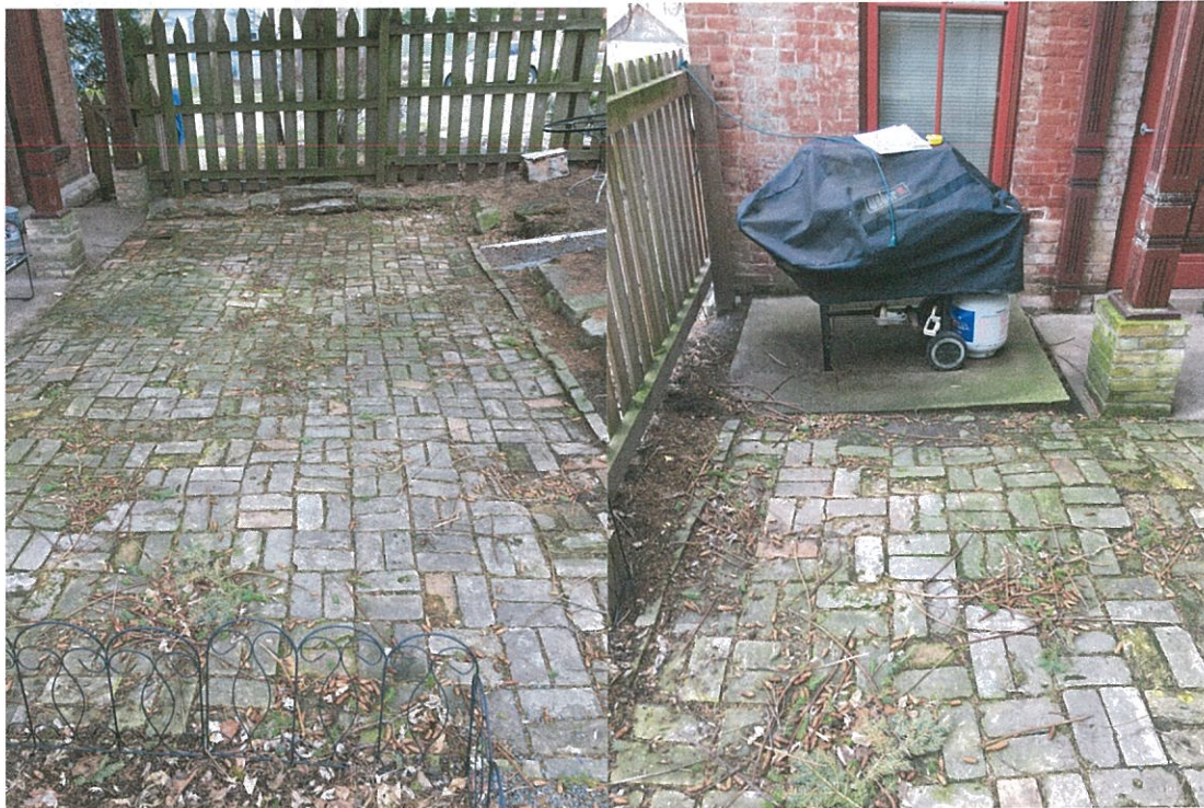
Existing Back Yard Patio and Concrete Stoop
