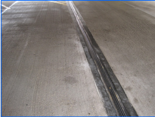
Elevated concrete floor slab
