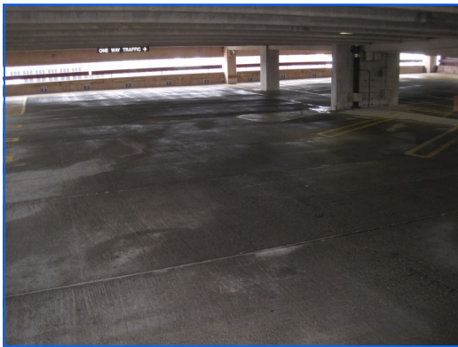
Elevated concrete floor slab
