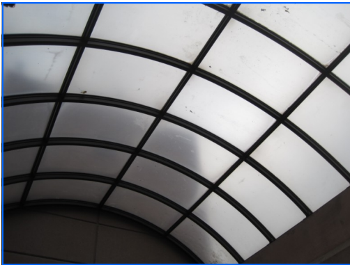
Part of skylight at south stairwell curtain wall
