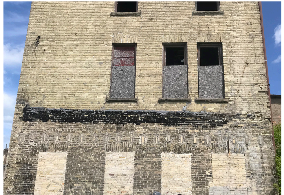
Existing back of building facade
