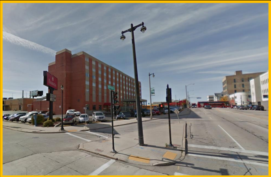
View from North 6 th Street and West Michigan Street
