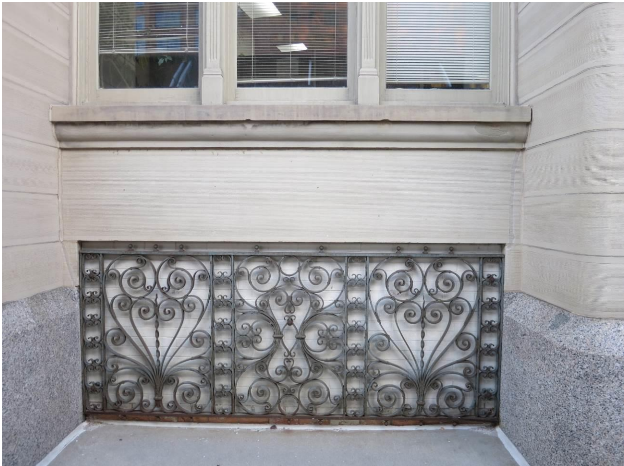
Typical Existing Wrought Iron Grille Work
