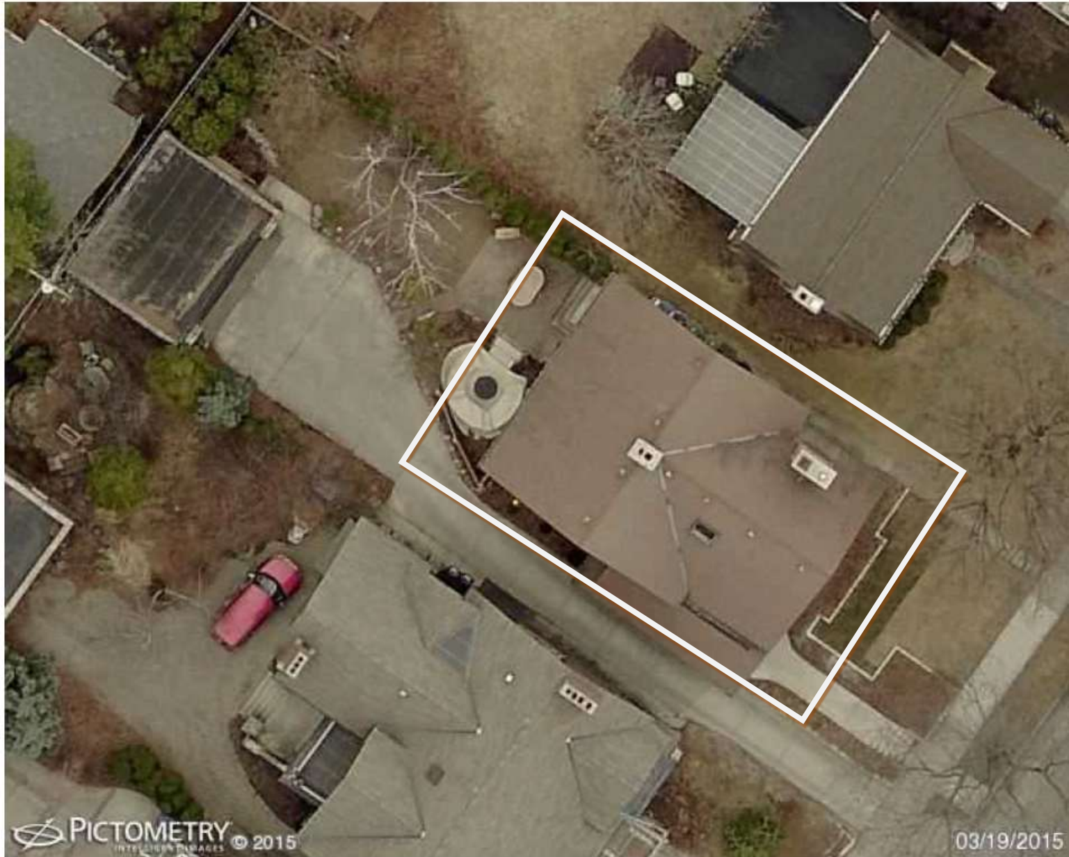
Aerial view of subject roof.
