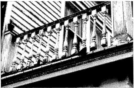
Upper guard rails to be rebuilt with new balusters. Fluted baluster posts to be retained and repaired and urn-shaped finials to remain. Deteriorated clapboards will be repaired/replaced with new wood siding to match.
