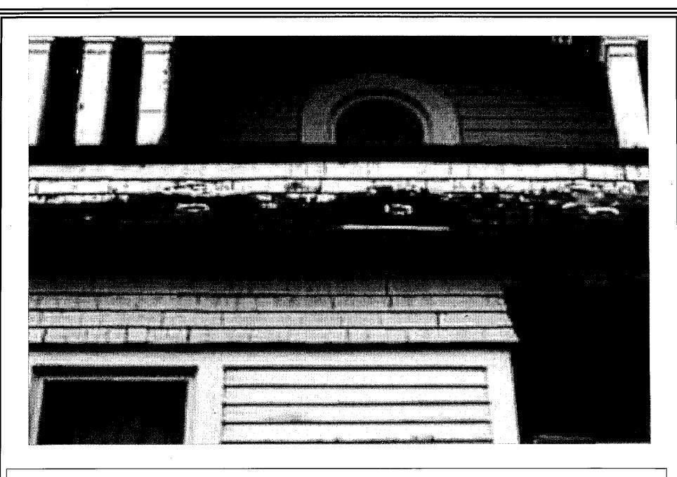
Deteriorated wood and fascia as well as shingles to be replaced as needed.
