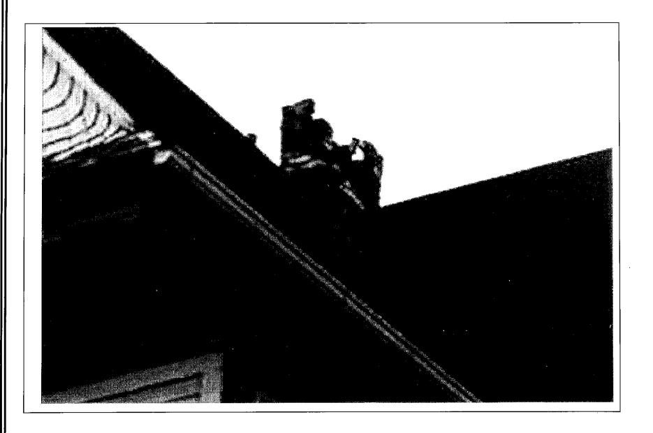
Repair deteriorated chimney using matching brick and appropriate mortar
