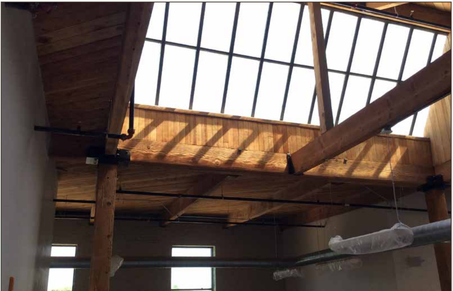
Third floor skylight.
