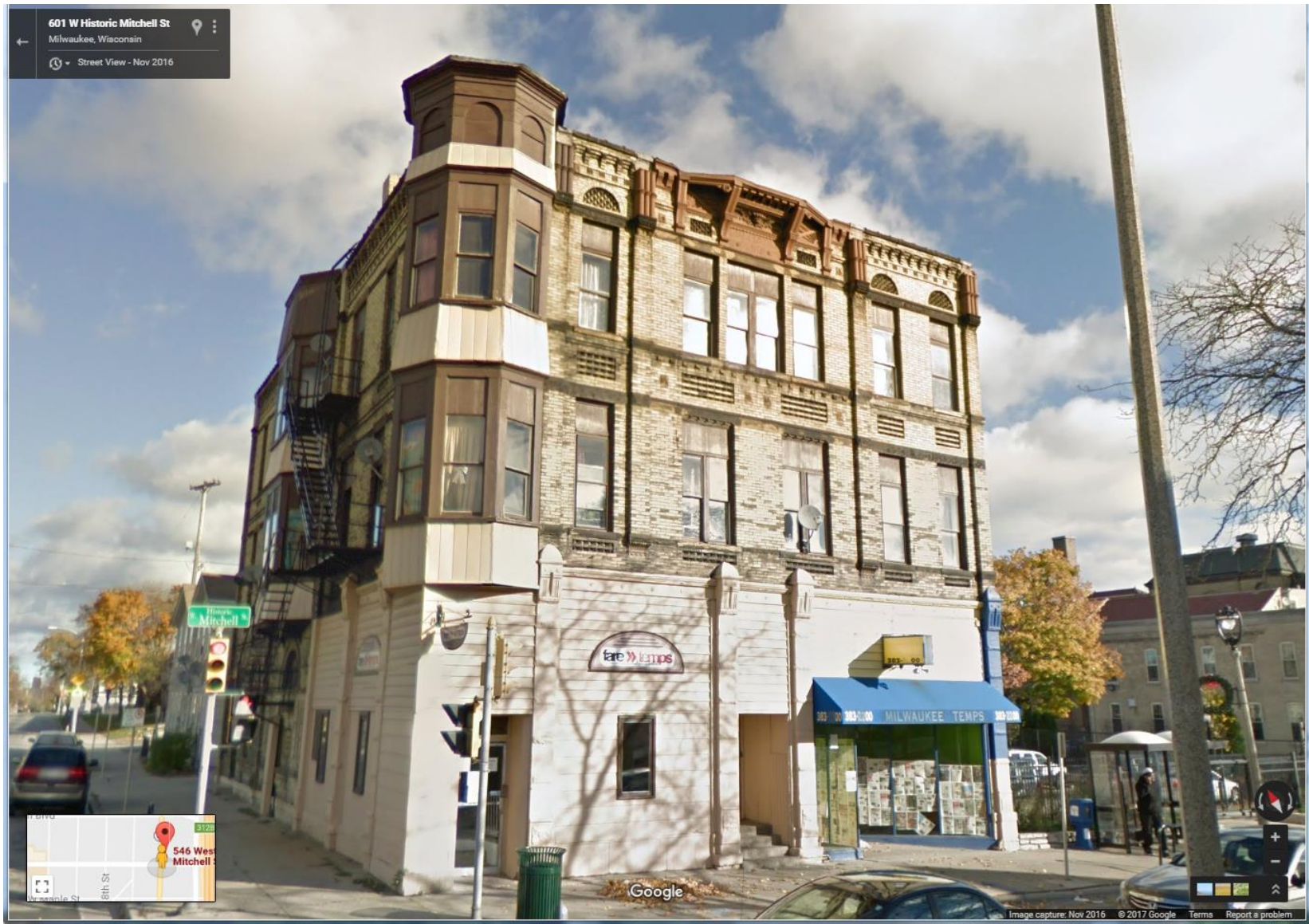
View of affected façade of building
