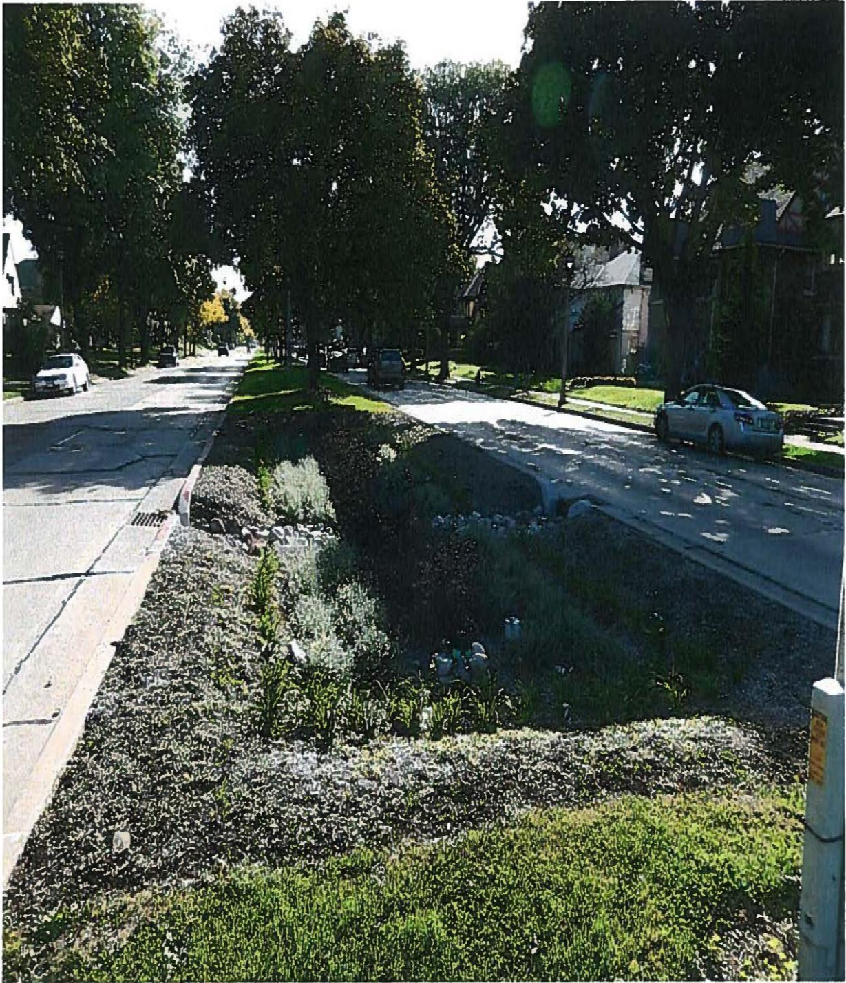
Finished Bioswale – Looking south
