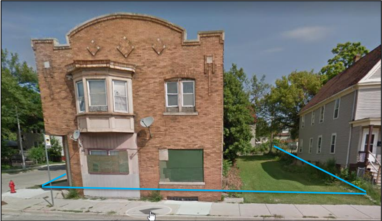
3610 & 3616 West Vliet Street (current conditions)
