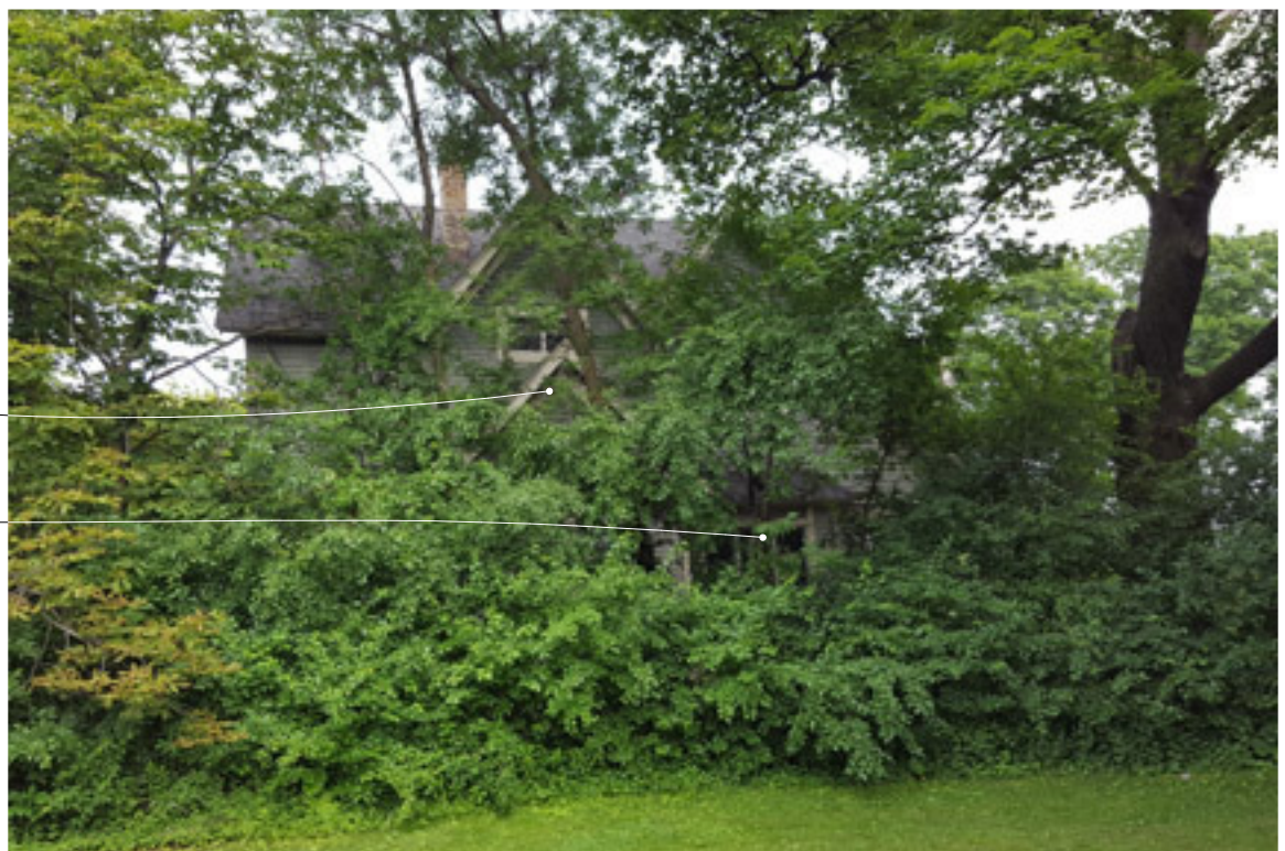
F SITE PHOTO
