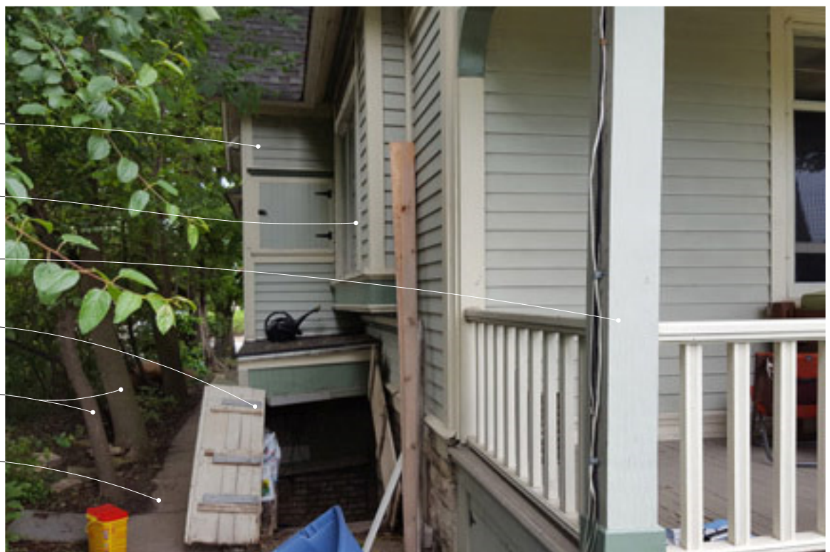
E SITE PHOTO
