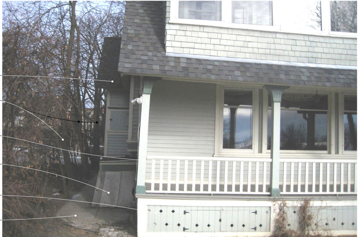
D SITE PHOTO
