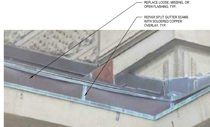
9 DETAIL @ ROOF CORNER FLASHING 1 1/2" = 1'-0"
