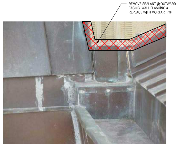
6 DETAIL @ INSIDE CORNER AISLE/TRANCEPT ROOF 1 1/2" = 1'-0"
