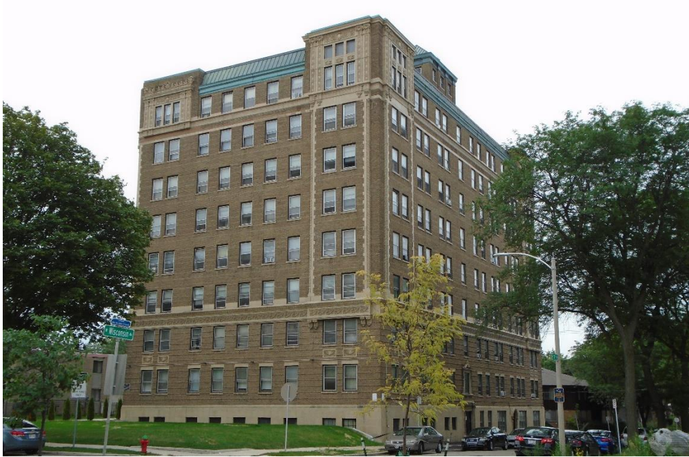
View looking southeast from W. Wisconsin Ave.
