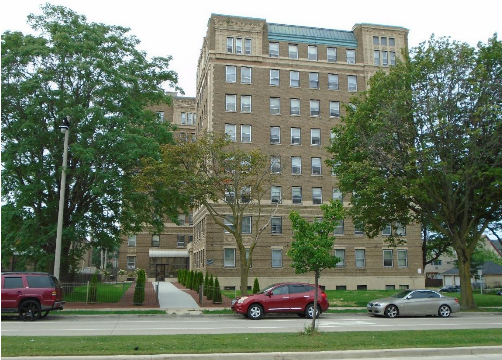
View looking south from W. Wisconsin Ave.
