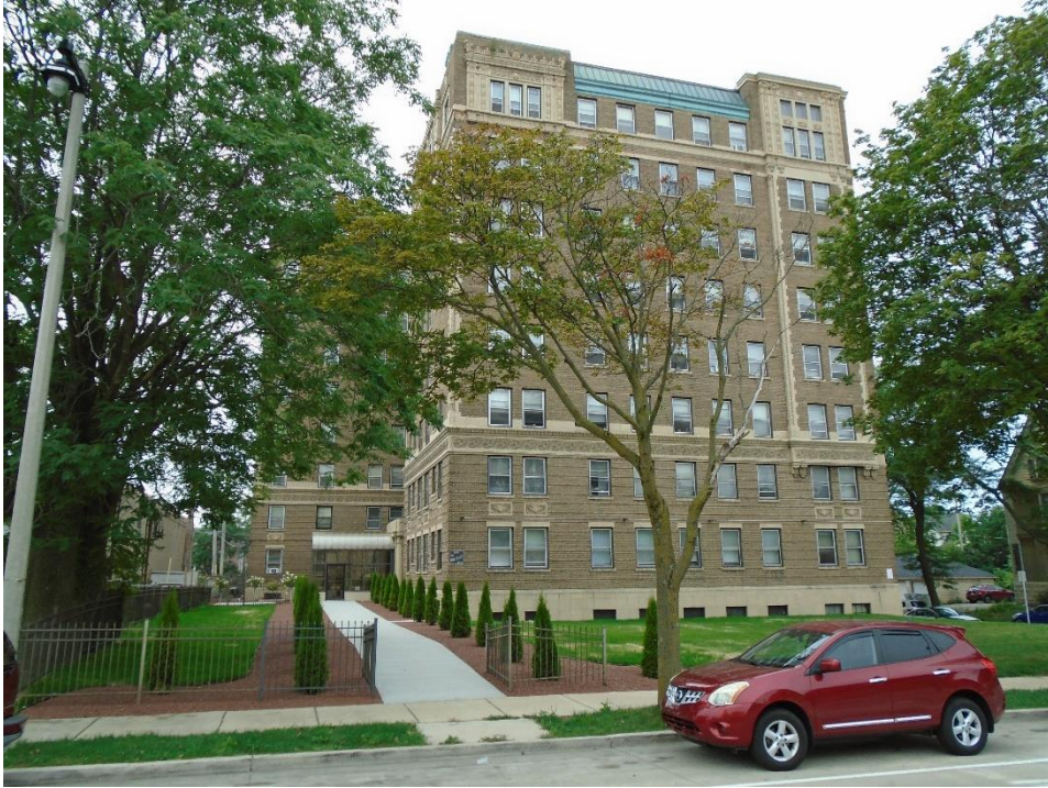
View looking south from W. Wisconsin Ave.
