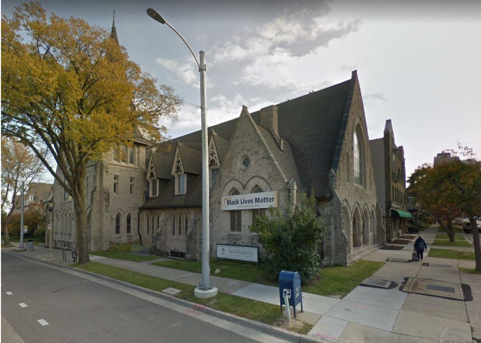
Location of existing monument sign at north facade
