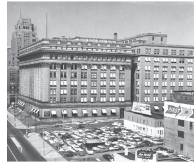
Current Home Office with 1932 addition, 720 E. Wisconsin Ave., 1914-present
