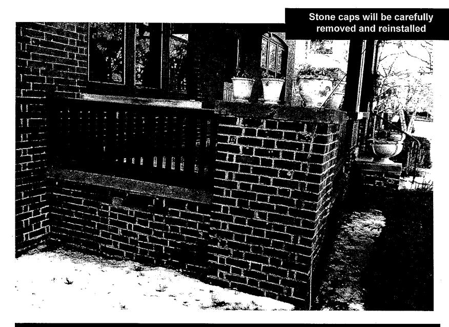
No change to design and mortar color, texture hardness, joint width and joint finish must match the original on the house.
