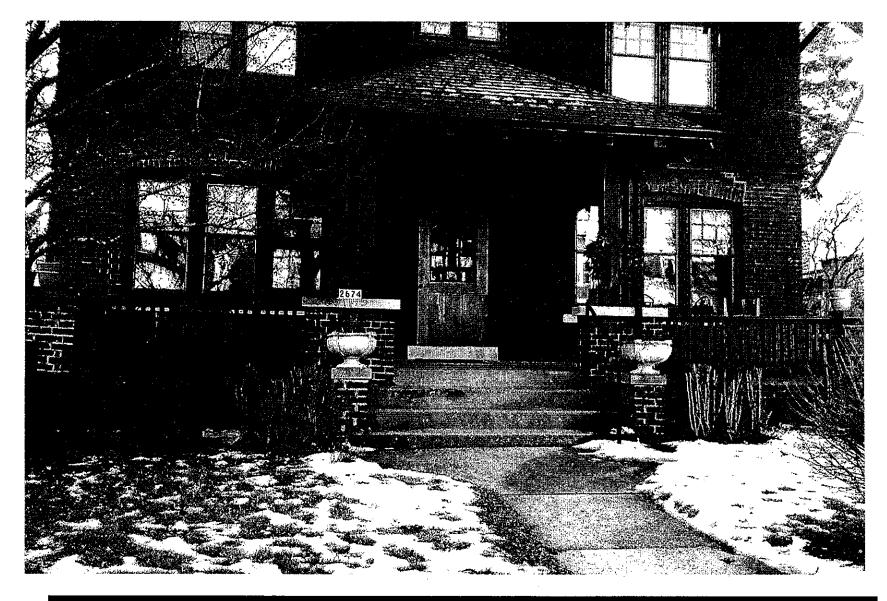
Rebuild Front Porch using salvaged brick and stone. Design will remain unchanged. New wood railings will match exactly the existing railings.
