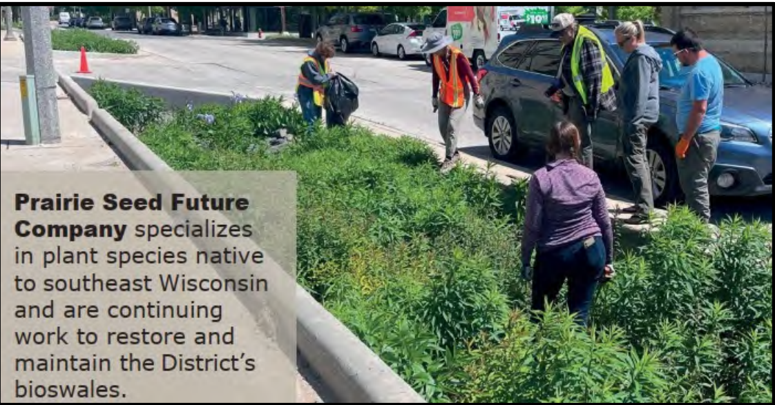
NID 1 – The Brewery Bioswale Maintenance
