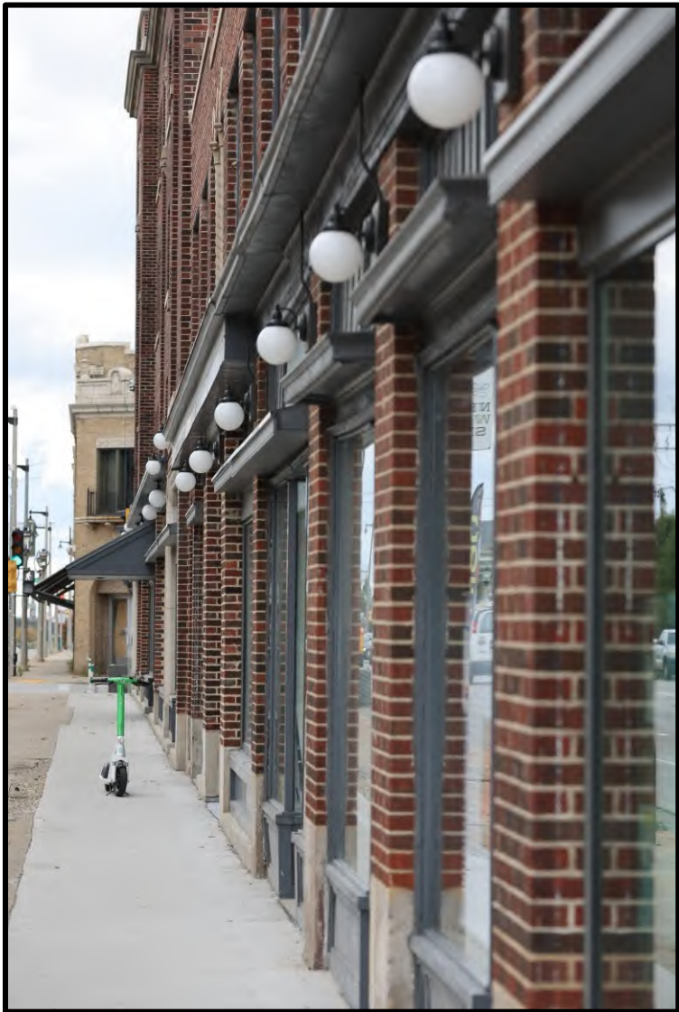
Concordia 27 building, located in BID 10, funded by Commercial Revitalization Grants.
