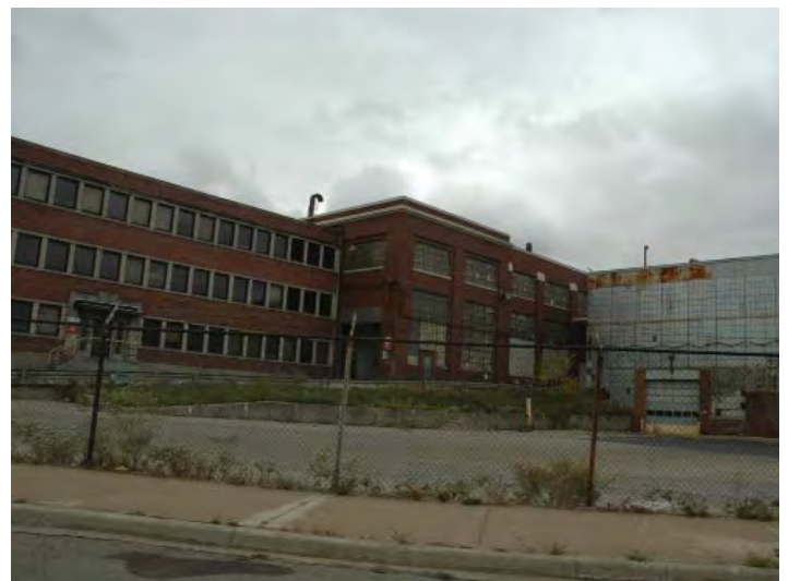
Existing conditions are mostly impervious, particularly at the Century City site.
