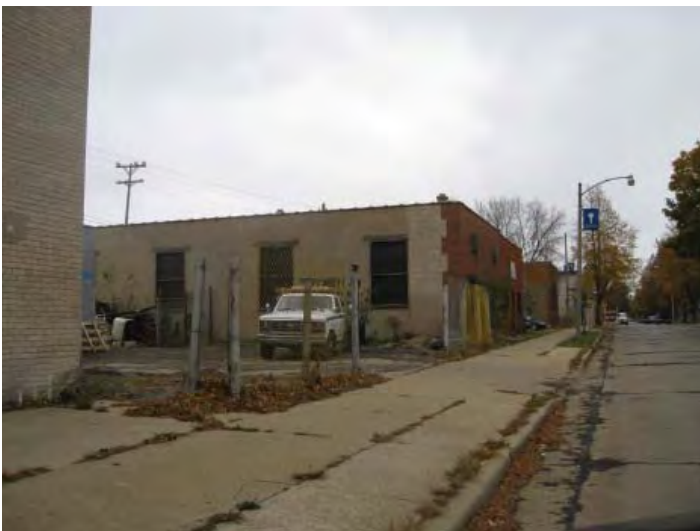
Many long-time active industrial uses, particularly on 30th St., are insufficiently buffered from the surrounding residential area.
