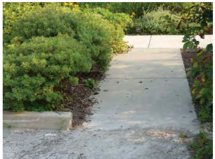
Paved areas can be designed with soft edges or curb notches to facilitate stormwater flow to landscaped areas.
