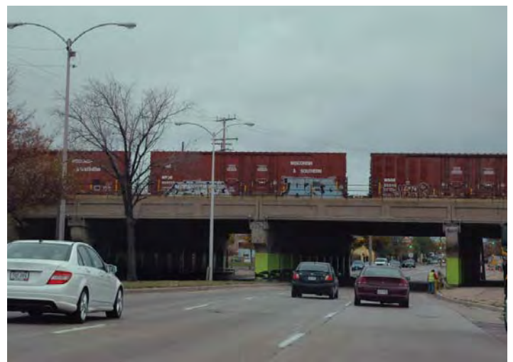
Viaduct at Capitol Dr.
