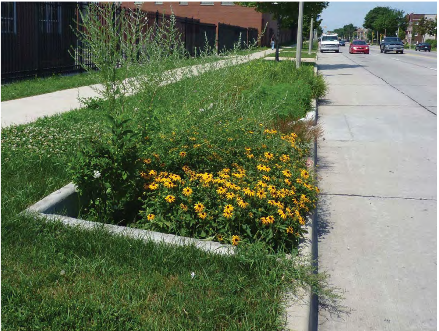
Bioretention area on 27th St., north of Capitol Dr.
