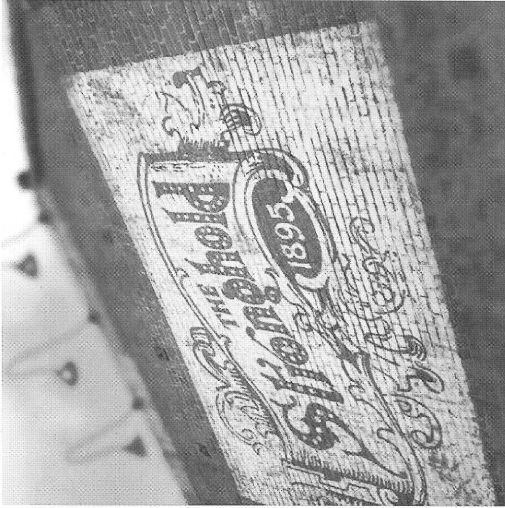
FACADE | GHOST SIGN BUILDING 23 | 1037 W. JUNEAU AVE.
