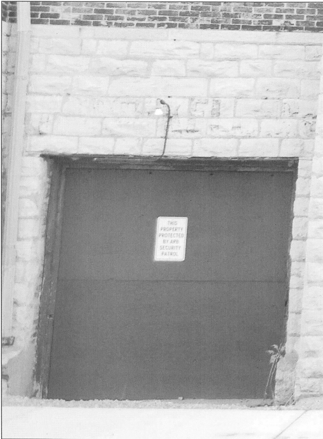
Image 8. The “Forstkeller” painted ghost sign over the west overhead door.
