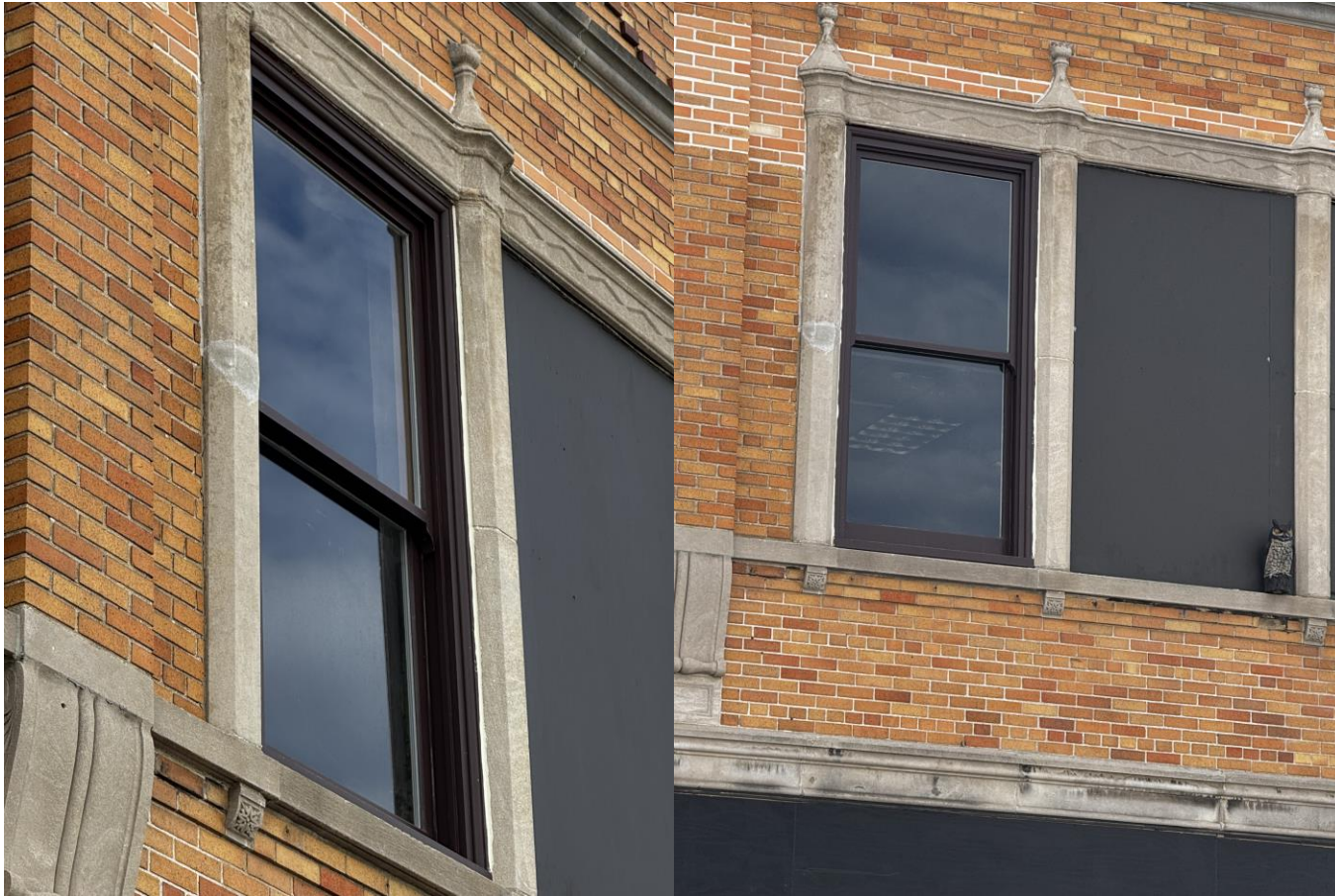
Mockup installation of proposed replica windows.
