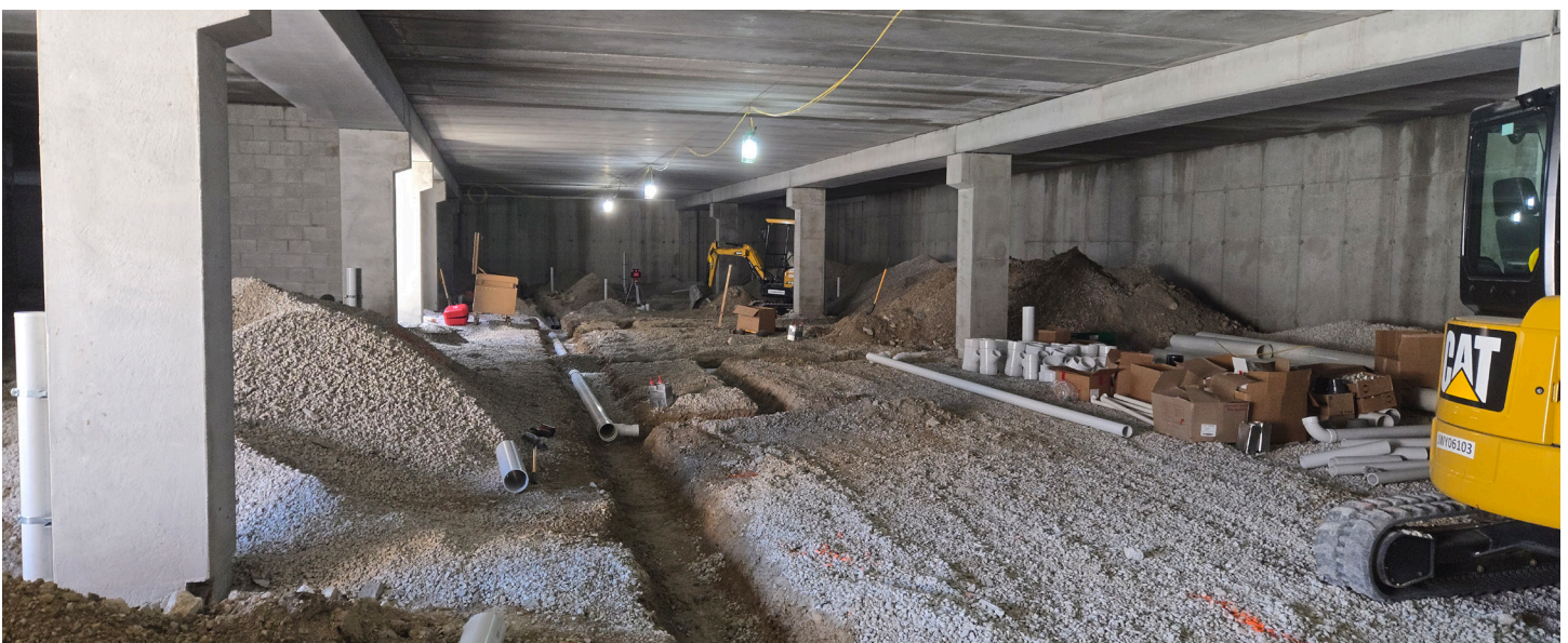
Some unground plumbing and electrical work being completed.
