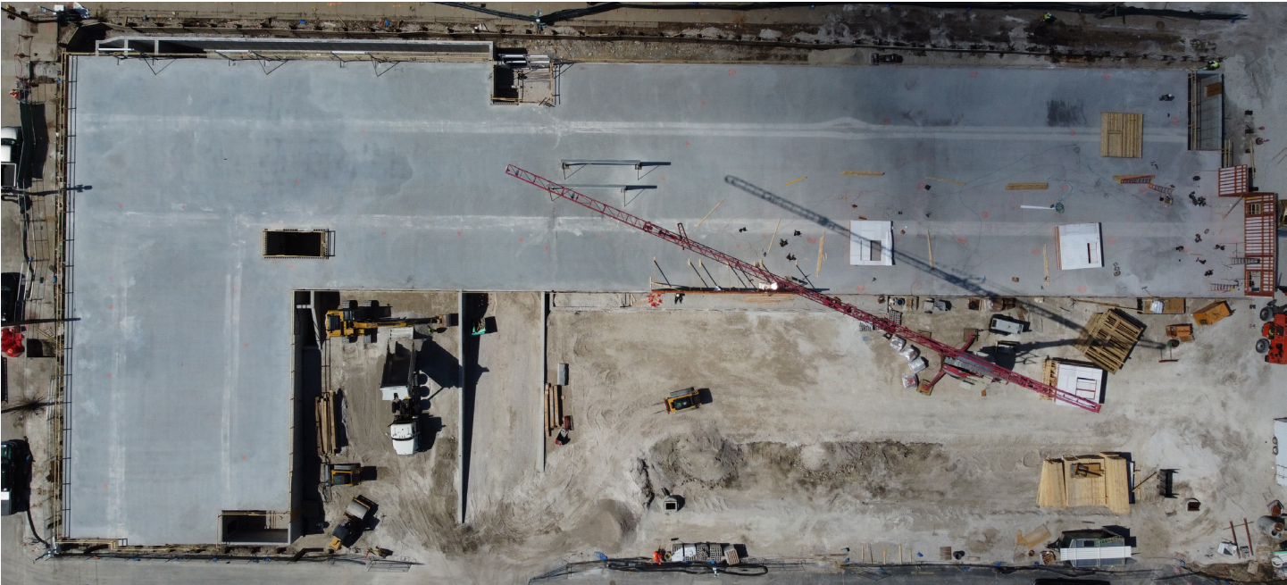
First-floor wall panels being delivered and installed on the first floor.
