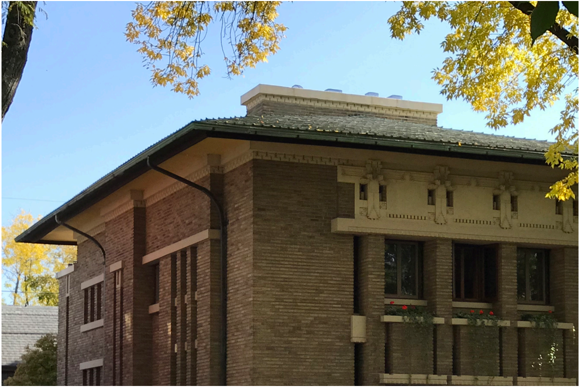
IMAGE 01: Photograph of chimney cap from Terrace Avenue.
