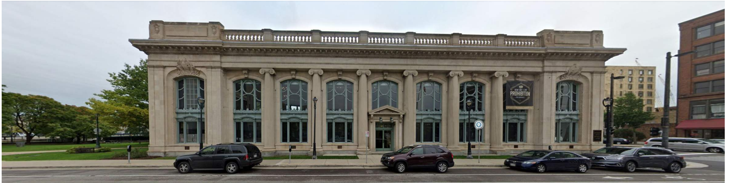
N. MLK JR. DRIVE | EAST SIDE OF STREET OPPOSITE SITE
