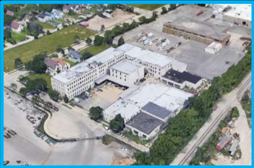
Aerial view looking northwest
