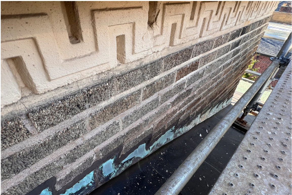
IMAGE 04: Photograph of stepped copper flashing at base of chimney.
