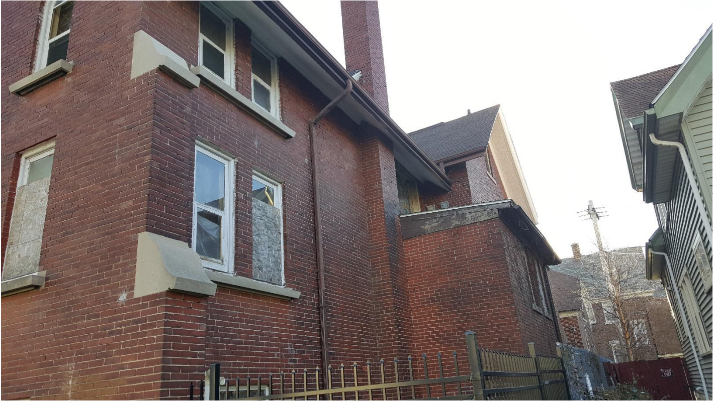
Fig.2 – Photo of West Elevation
