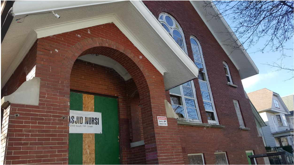
Fig.4 – Photo of North Elevation
