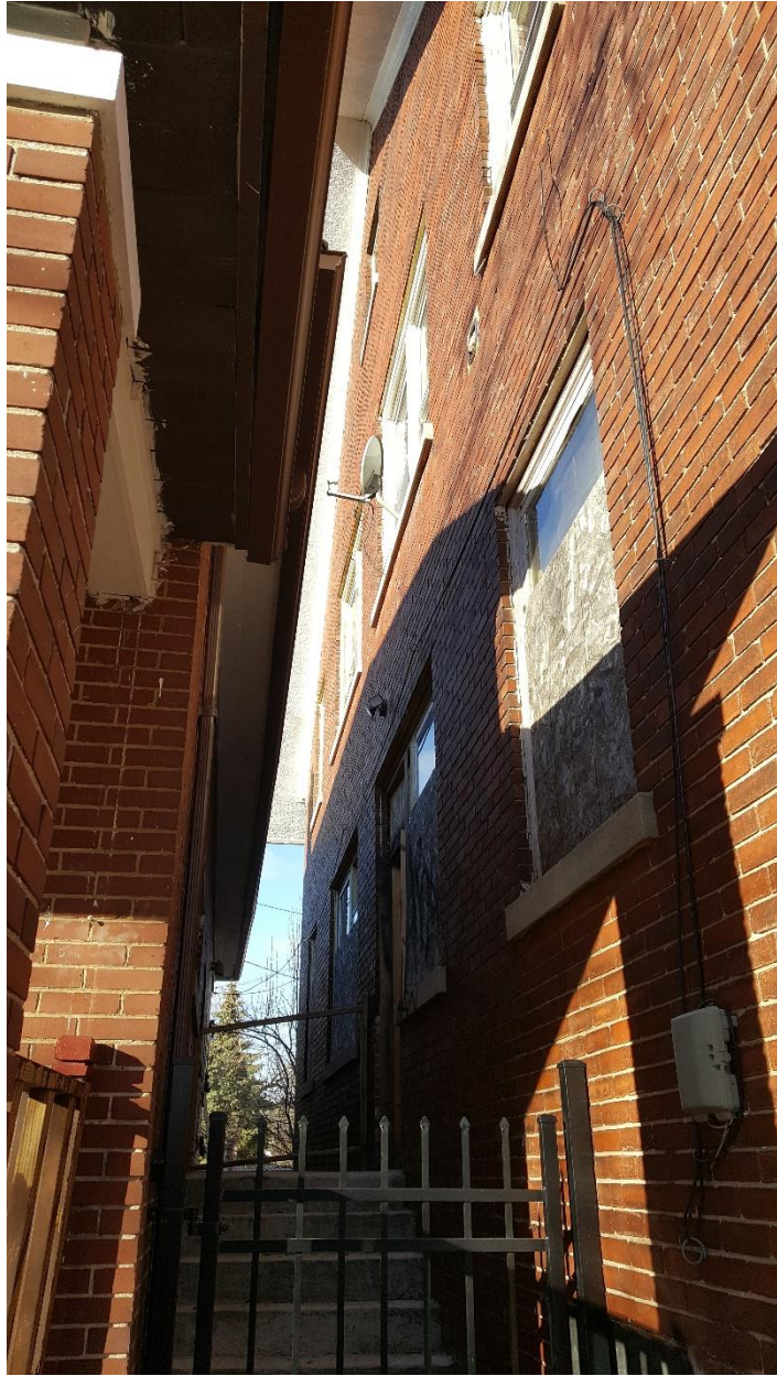
Fig.3 – Photo of South Elevation
