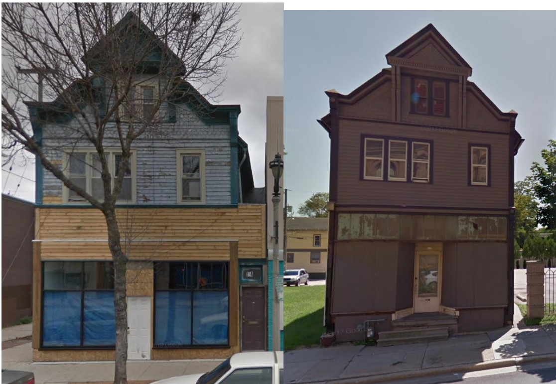
At left is 814-816 W. Historic Mitchell. At right is 515 W. Historic Mitchell. They are very close twins and explain what happens when you bring down the level of the entrance. At Mr. Salinas' building the 1938 remodeling brought the storefront down to grade. Since the interior floor was higher than the sidewalk (as seen in near twin) the deep recessed entry was created which actually ramped up to the entrance. The deep recessed area held display windows and was intended to draw customers to the entrance. It also brought down the transom which left an awkward area above, covered by metal or wood panels. The decorative headblocks/brackets at each end were removed.
