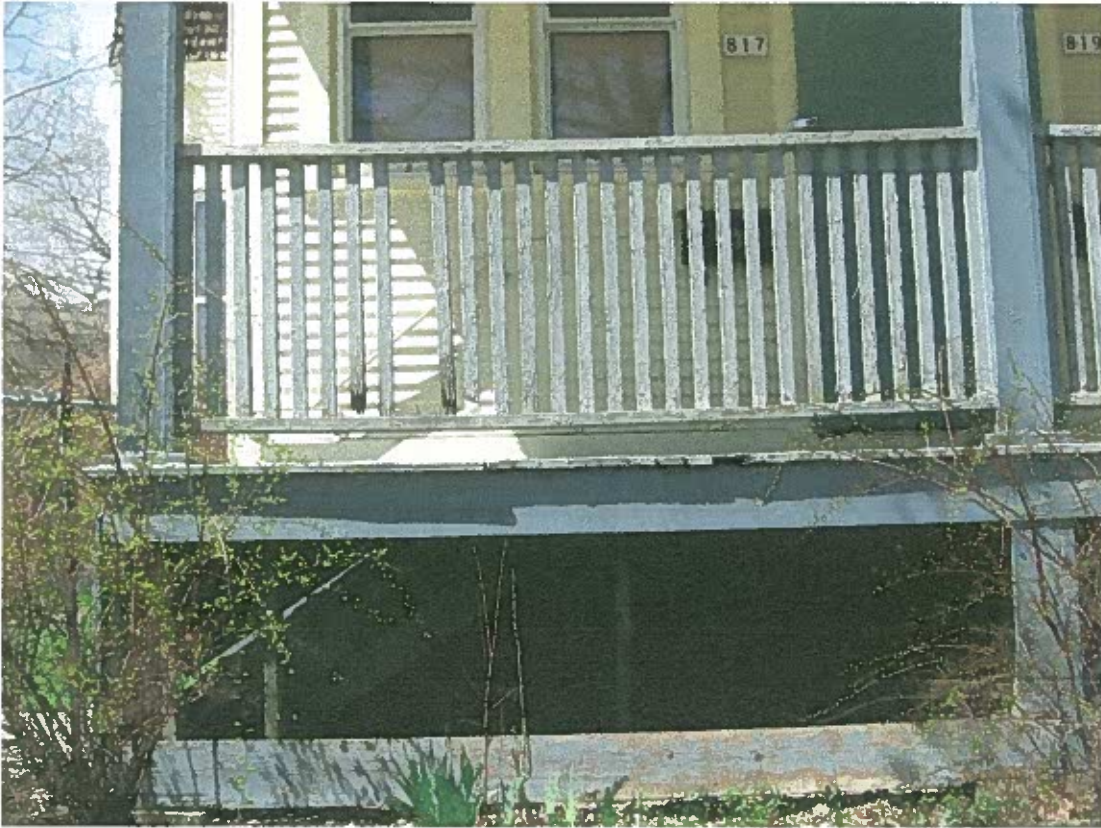
5. Front Porch (East Elevation) Columns, Railing, and Skirt
