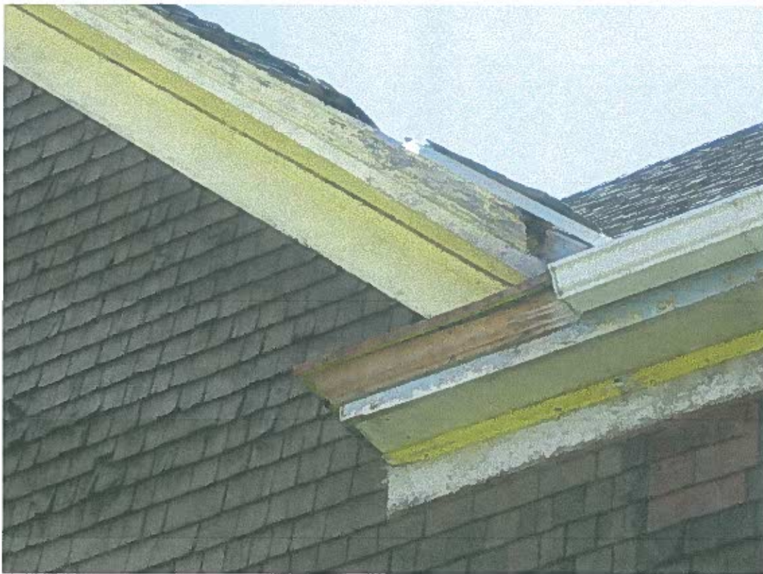
4. Wood Shingle Rear Gable (West Elevation) w/ eave connection & K-style gutter
