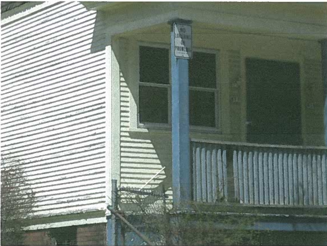
6. Front Porch (East Elevation) Column and railing
