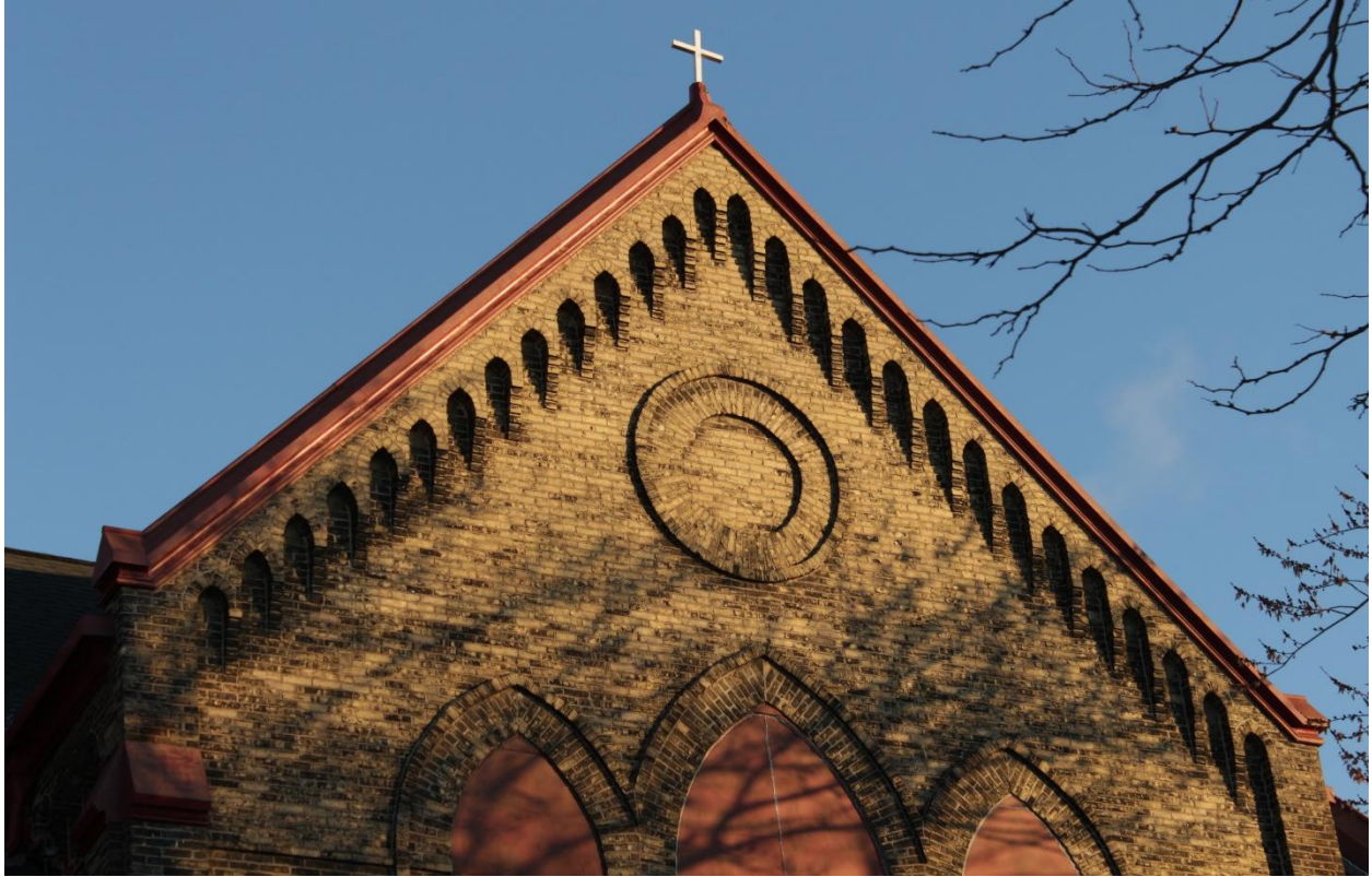
Figure 14: Gothic style brick corbelling on gable wall, 2025.
