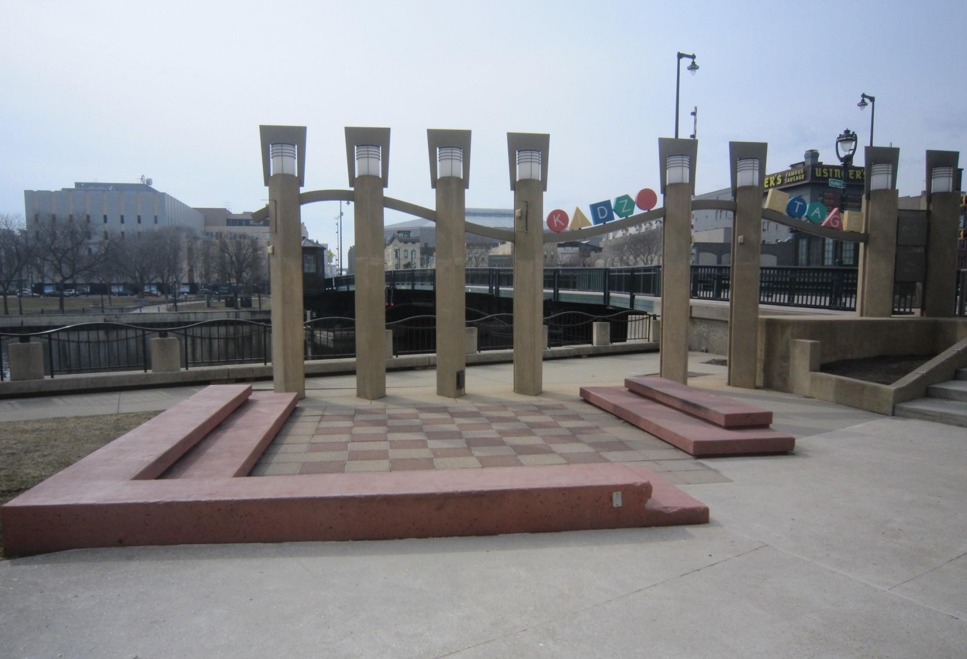
Kidz Stage Riverfront Theater; Opening 2000 Kahler Slater Architects
