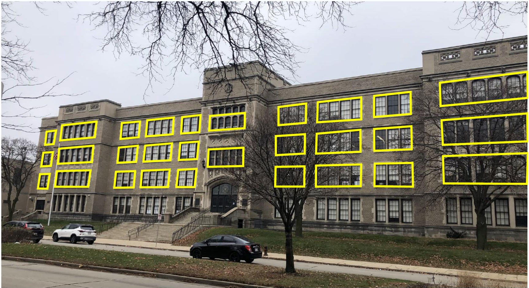
Washington: East Elevation Sherman Blvd
