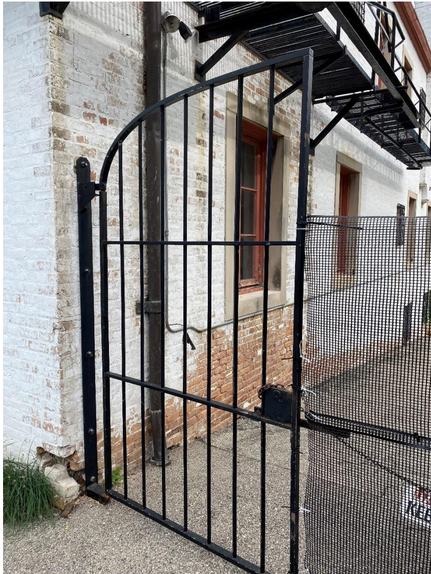
Existing gate and replacement gate
