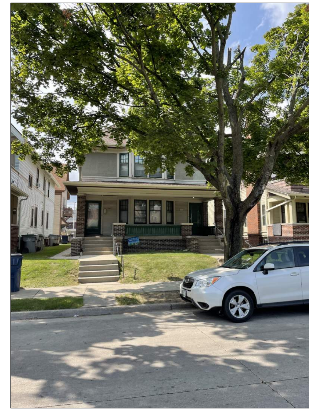
4 PHOTO FROM STREET SCALE: NONE
