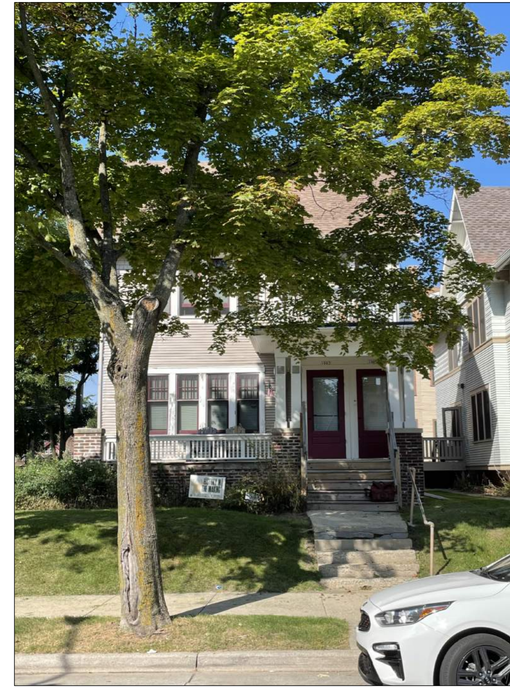
3 PHOTO FROM STREET SCALE: NONE
