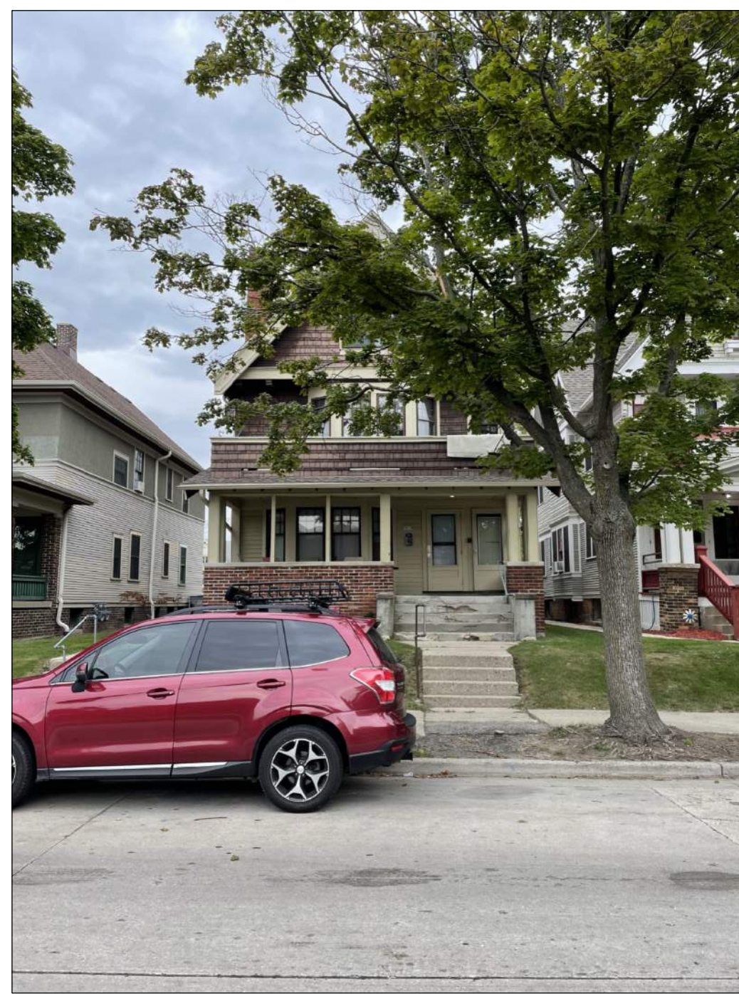
4 PHOTO FROM STREET SCALE: NONE
