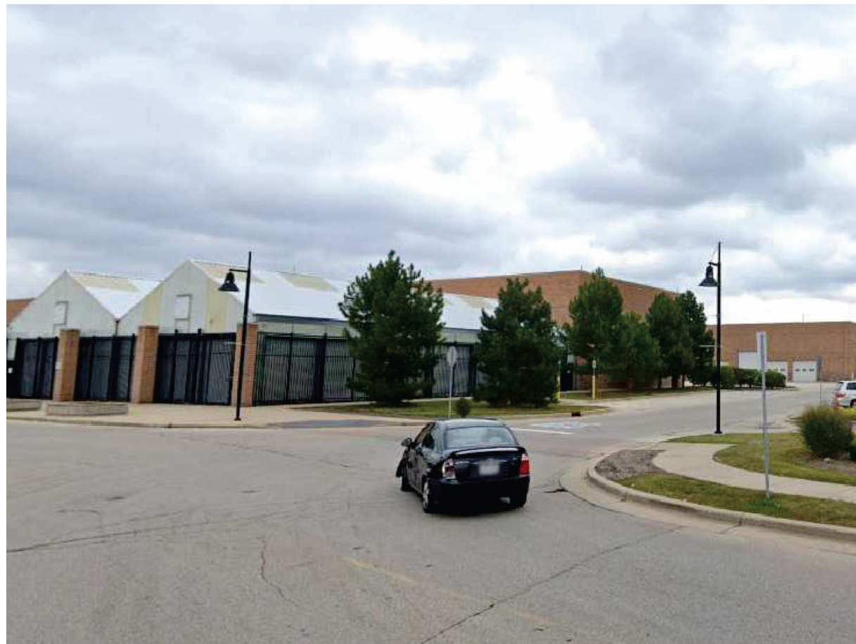
NORTHWEST SIDE OF BUILDING - EXISTING GREENHOUSES
