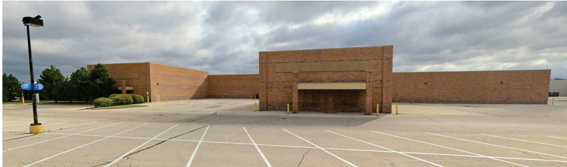
WEST SIDE OF EXISTING BUILDING
