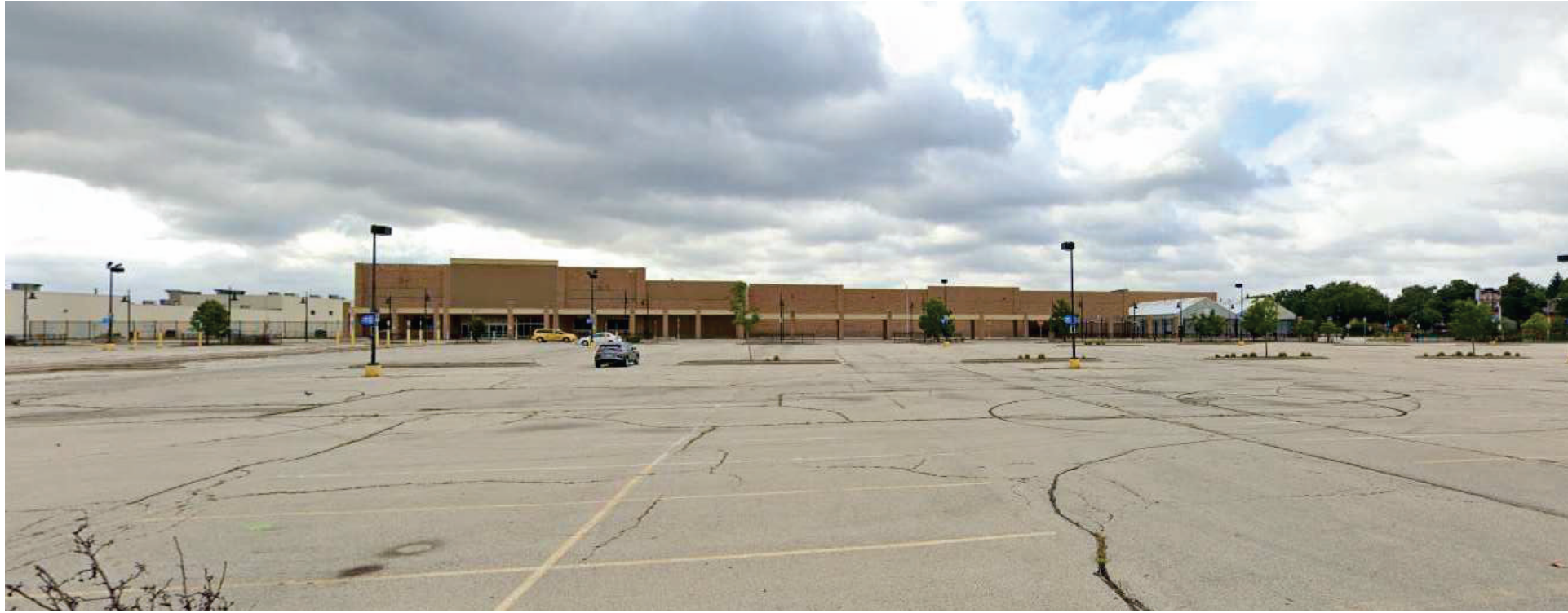
NORTH FACE OF EXISTING BUILDING
