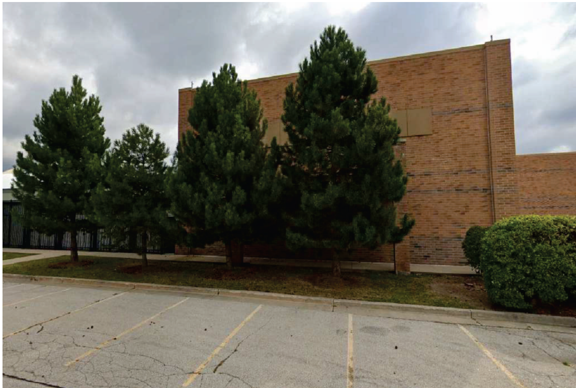
WEST SIDE OF EXISTING BUILDING
