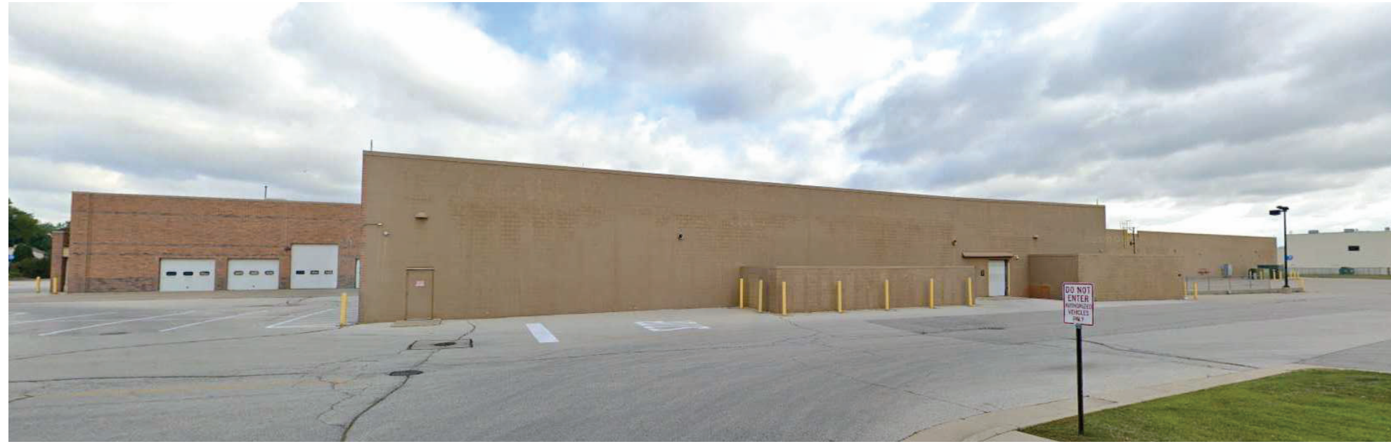
SOUTH SIDE OF EXISTING BUILDING
