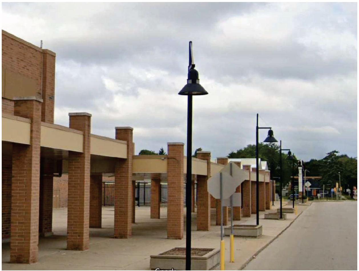
NORTH SIDE OF BUILDING LOOKING WEST
