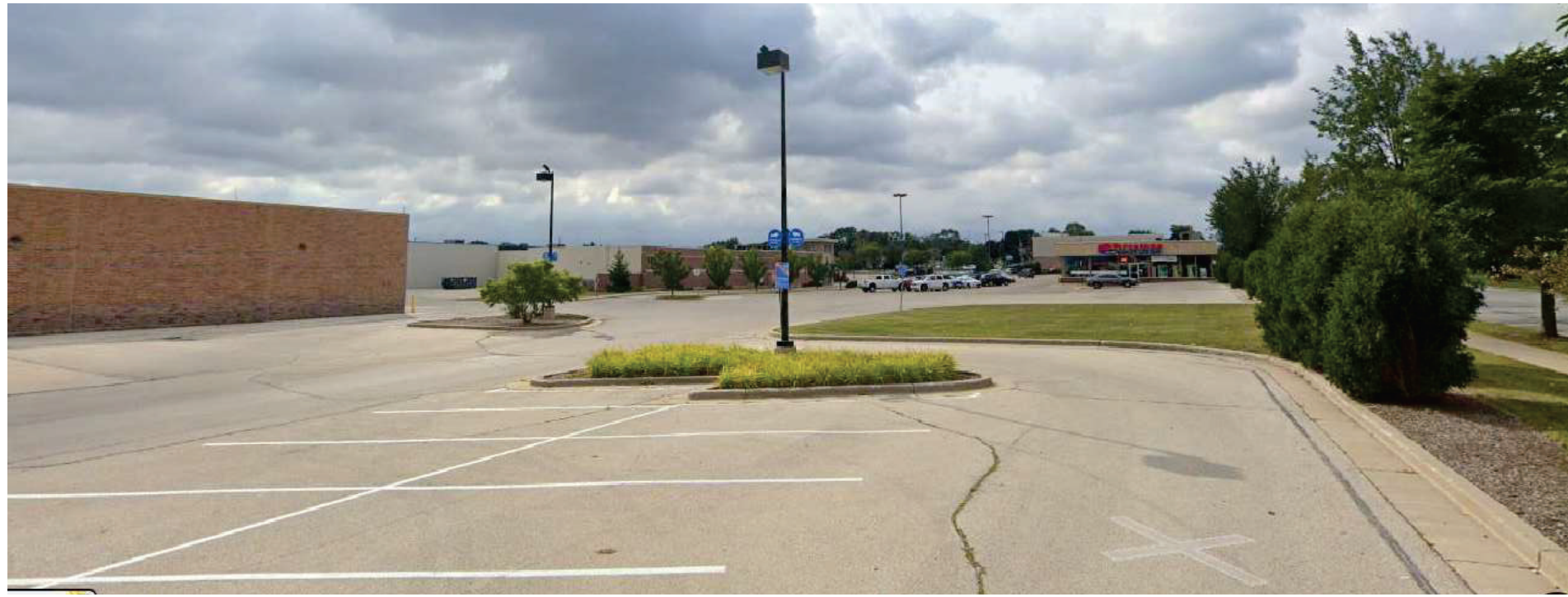
SOUTHWEST CORNER OF EXISTING BUILDING
