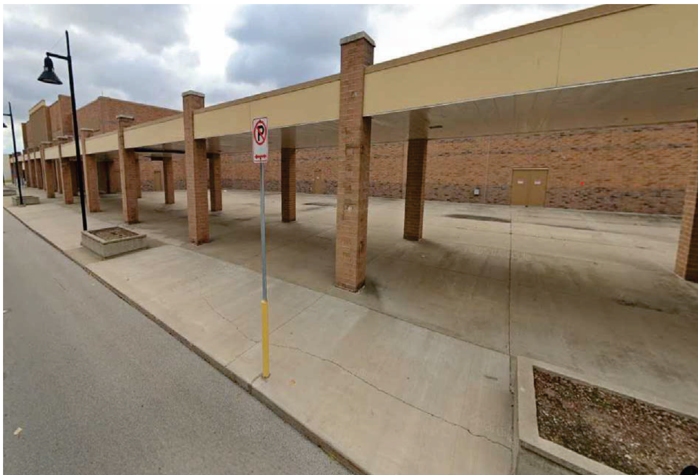
NORTH FACE OF BUILDING - COLONNADE
