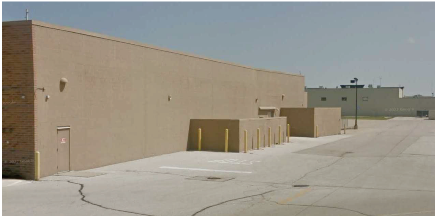
SOUTH SIDE OF EXISTING BUILDING
